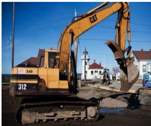
Road Construction at the lighthouse. Photo courtesy The Herald
