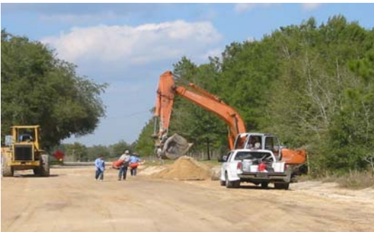
Georgetown Shortcut – Work in Progress
