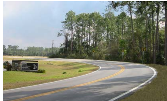
CR309 – Widening and Resurfacing
