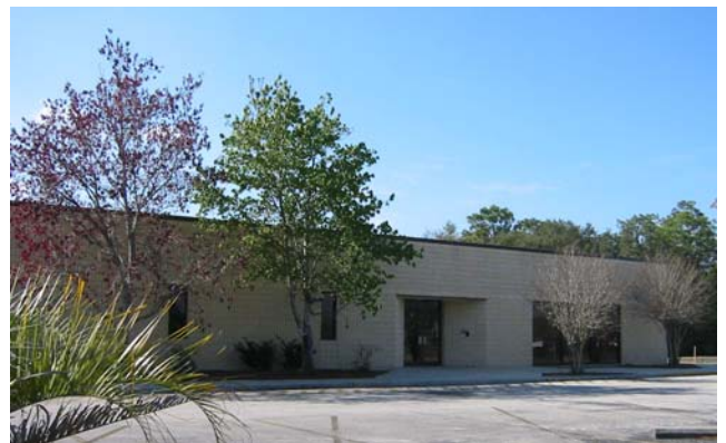
The new Putnam County Emergency Operations Center. Formerly the Bell South telephone center, the building has 20,000 SF of useable space. Its central location on Hwy 19 near Highways 17, 100 and 20 should make it the ideal location when the need arises.
