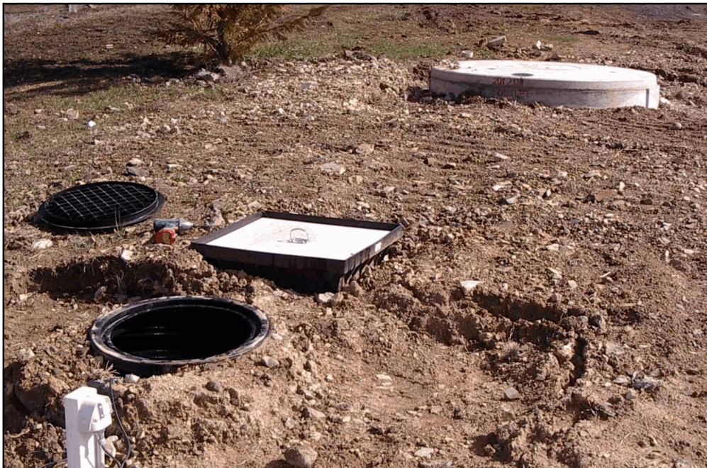
Figure 8: Septic tank flows into a filter tank, then a pump-well
