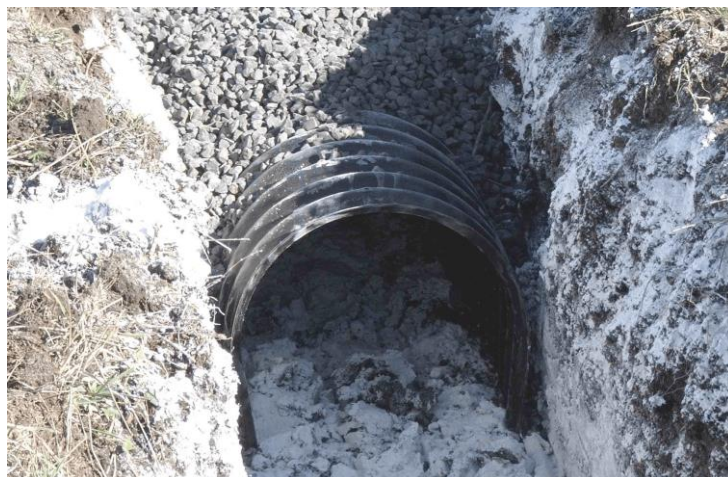
Figure 14: Lime spreading in trench
