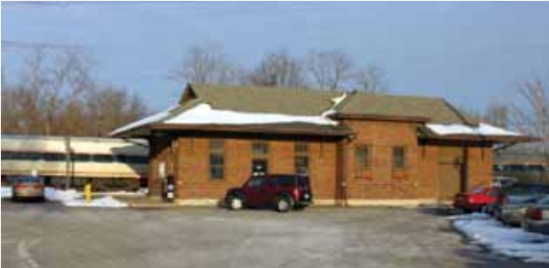
Current Amtrak Station, Alton, Illinois
