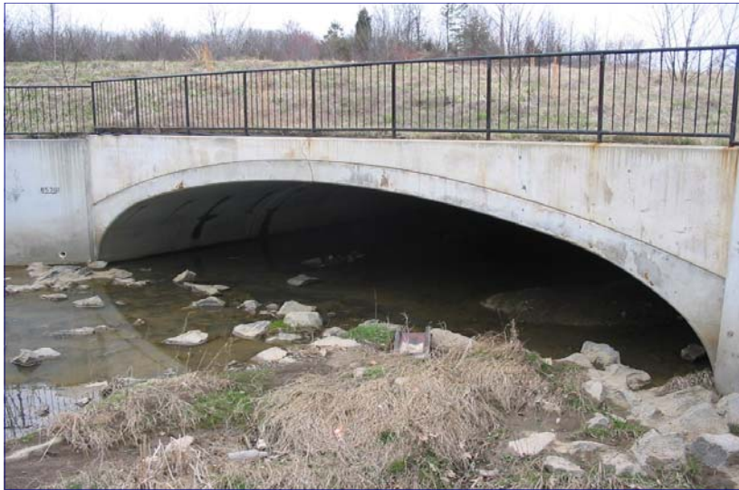
IMPACTS 3, 4, 5 - Bottomless culverts with scour protection.
