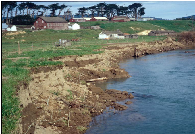
An eroding bank on the lower Garcia was causing loss of land on the Stornetta Brothers Ranch below Hwy 1 in 1995. Photo by Craig Bell.
