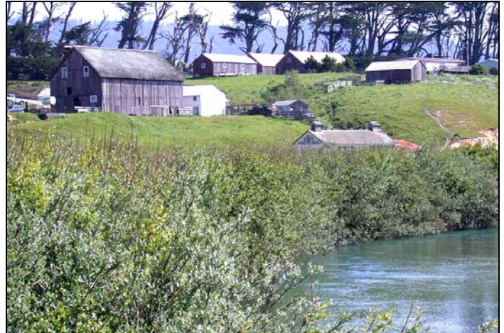
This is the same site as at left, in 2003, showing a fully restored bank that provides protection from erosion and forms excellent aquatic habitat. Photo by Craig Bell.
