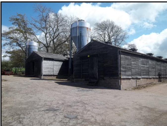
View of two main poultry sheds and feed bins
