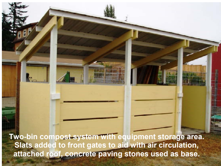
Pressure treated wood walls, attached roof, concrete apron and base.
