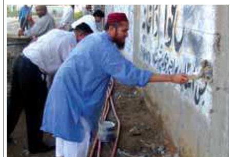
Removing of wall chalking
