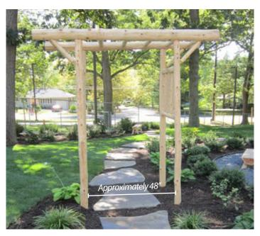
Narrow accessible route beneath Rustic Arbor to a width greater than 36 inches for a distance of 60 inches or less. The remaining accessible route should measure 60 inches.
