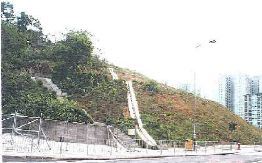
General View of Northern Side of the Slope (Date: 18 April yyyy)
