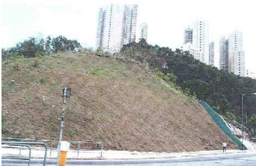
General View of Western Side of the Slope (Date: 18 April yyyy)
