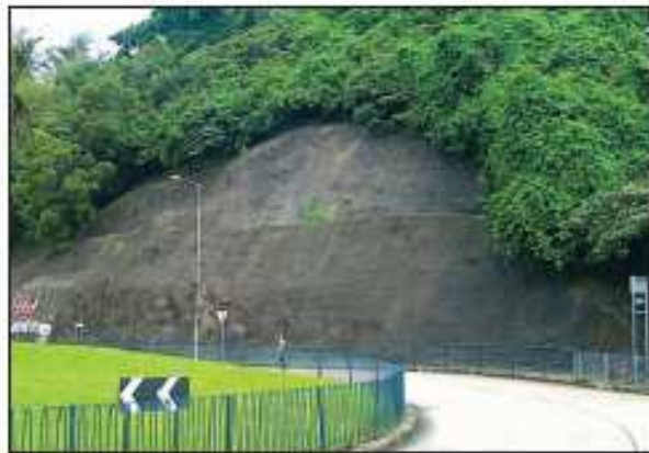
Slope before upgrading works (2001)
