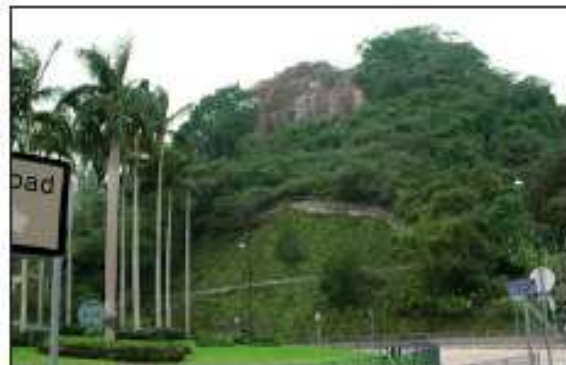
2 years after slope upgrading works (2007)
