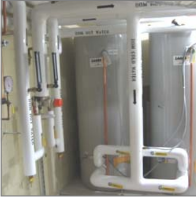
Domestic hot water boilers—Berksire, Kent, Wharfedale
