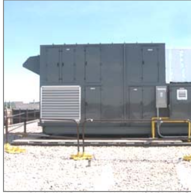
170 Kent Street—Make-up air system
