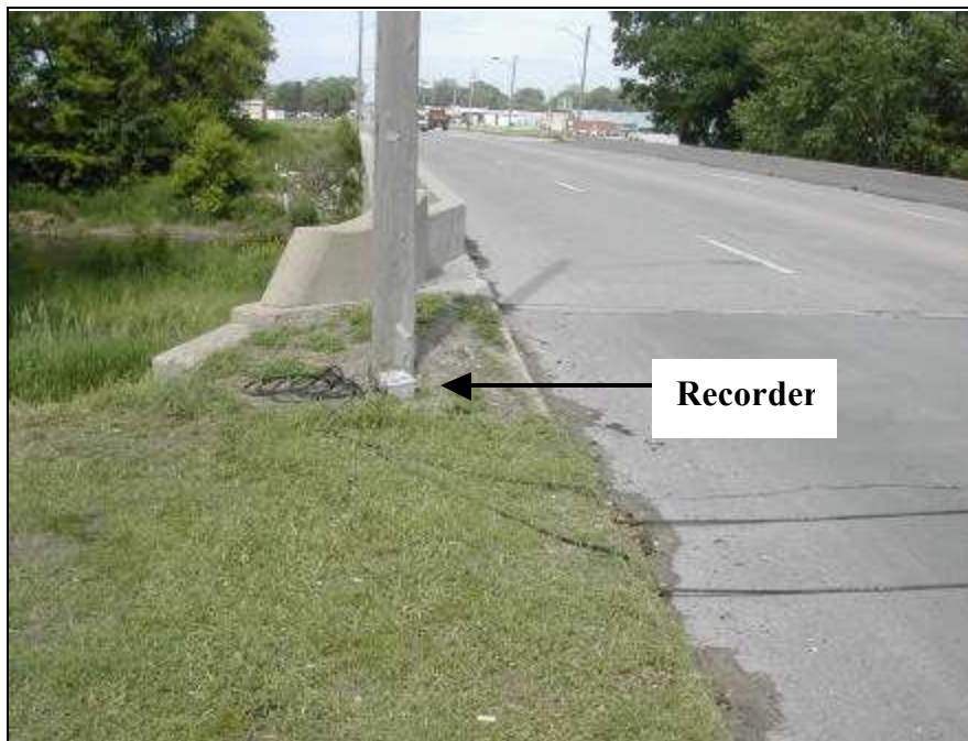
Figure 2.8. Road Tubes and Recorder
