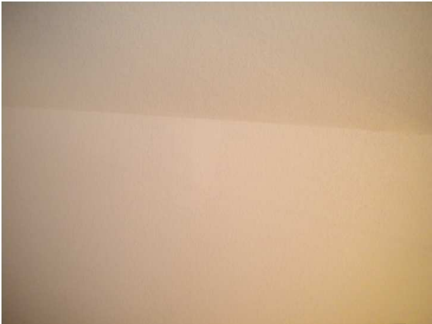
View of Ceiling@ Kitchen/Dining
