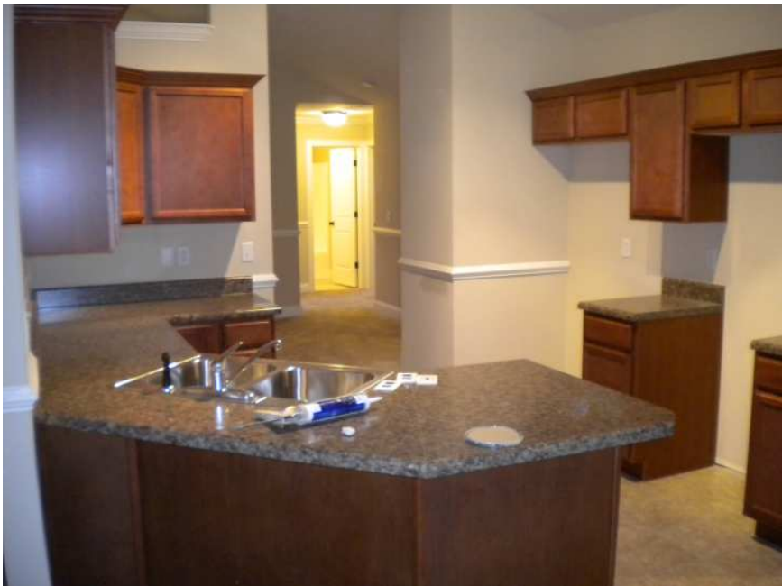
View of Kitchen
