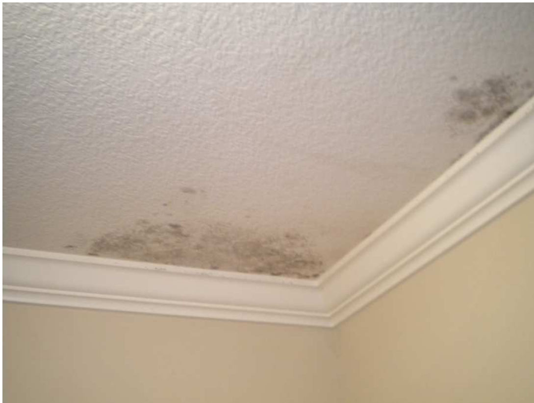
View of Ceiling@ Foyer
