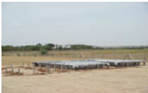
Illustration 9. Spirulina tanks. On the left, there are the concrete pillars where the frame and the tarpaulin have to be assembled. The other two tanks are ready for the Spirulina production.
