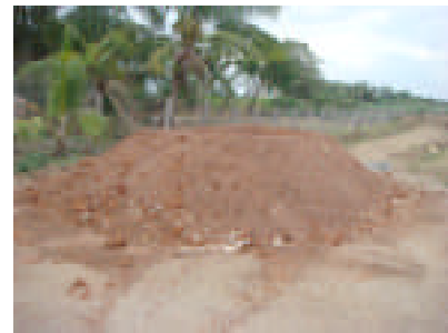
Illustration 7. The soil for the temporary water tank.
