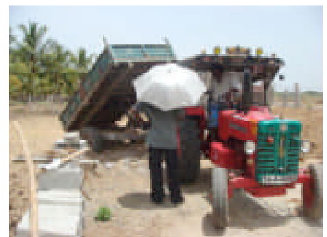
Illustration 3. A truck unloads another load of soil for the levelling.
