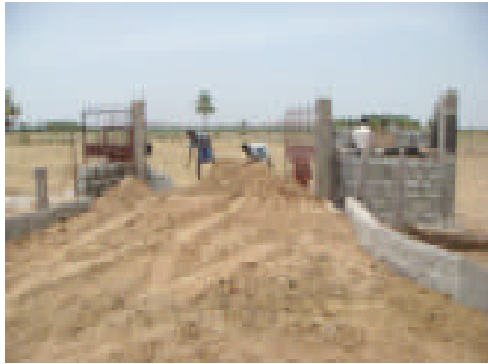
Illustration 4. The soil, which had to be added at the main gate to level the land with the road.
