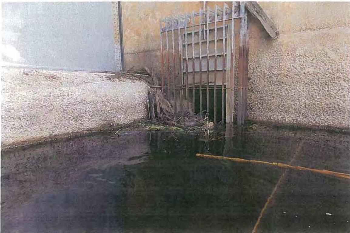
Upstream - South Bay, Upstream Face of Wier
