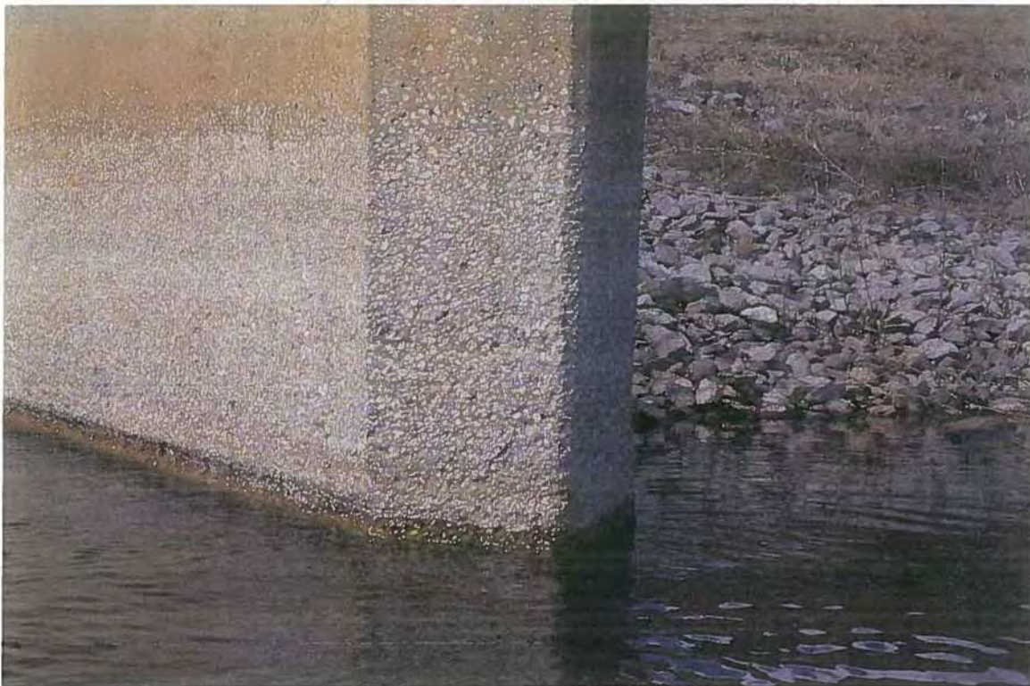
Downstream - North Wall Abutment. Steel Sheetpile Wingwall Under Water.
