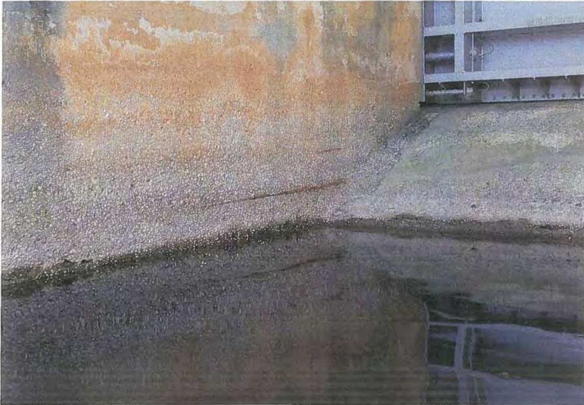
Downstream - South Bay Wall Near Spillway. Note Reinforcing Steel.
