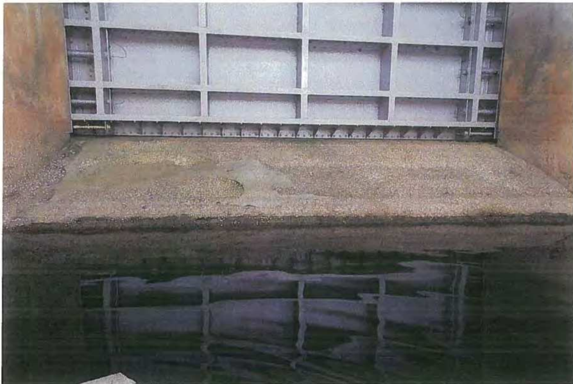
Downstream - South Bay Spillway
