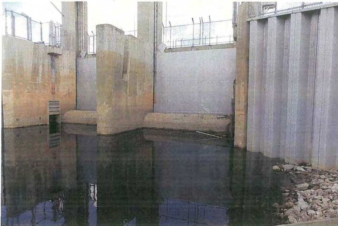
Upstream - North Bay Wall, Interior Wall with South Wingwall
