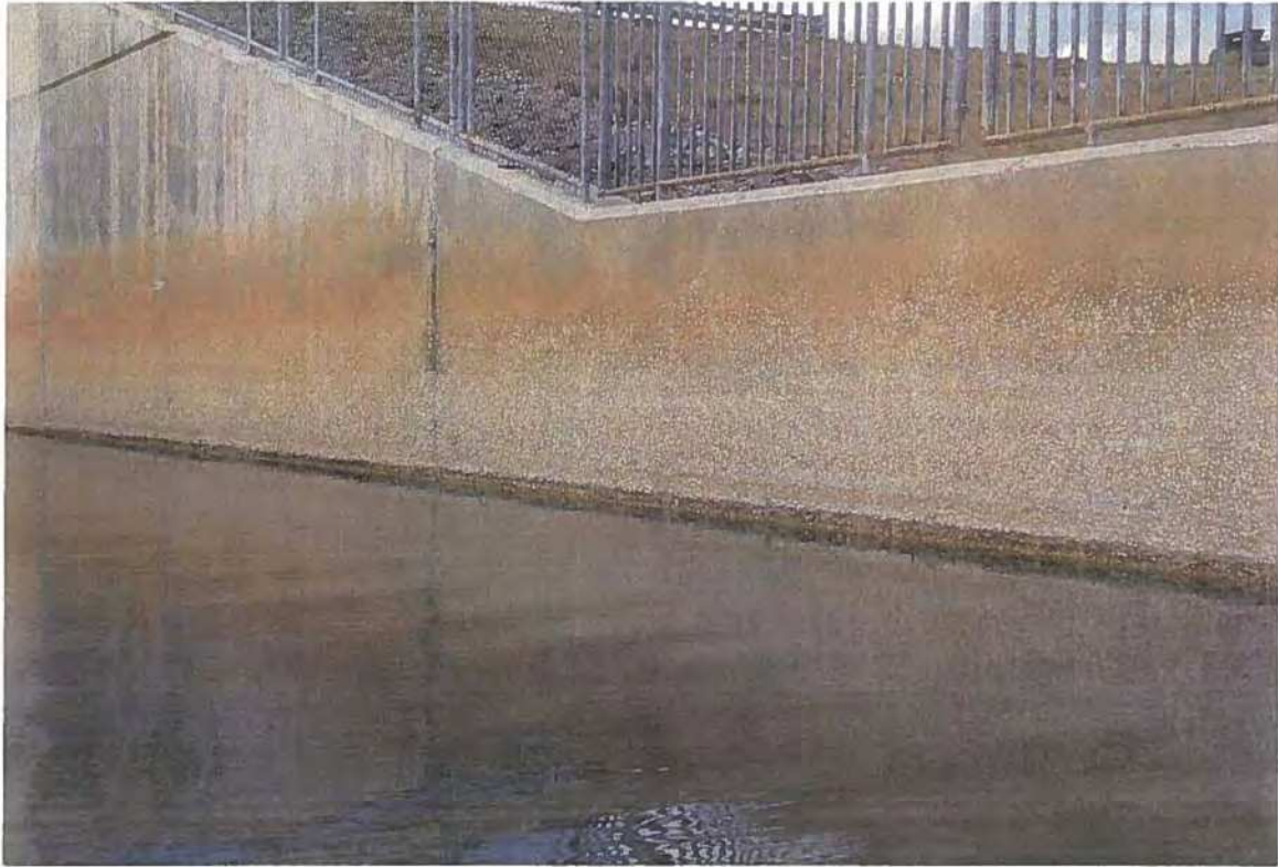
Downstream - North Bay Wall
