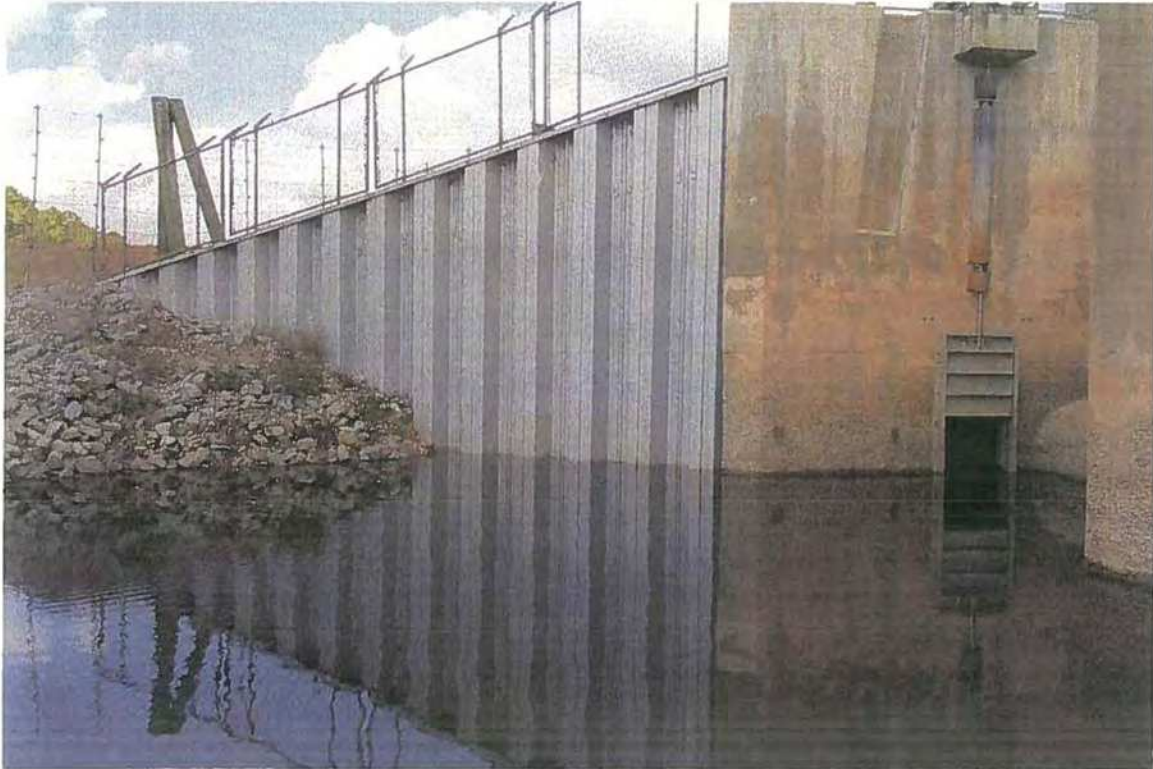
Upstream - North Wingwall / Bay Wall
