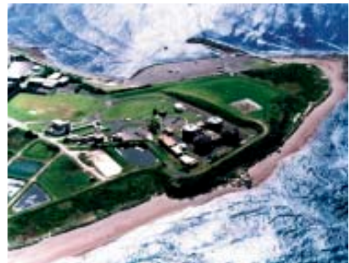
The existing Wollongong (LEFT) and Bellambi treatment plants
