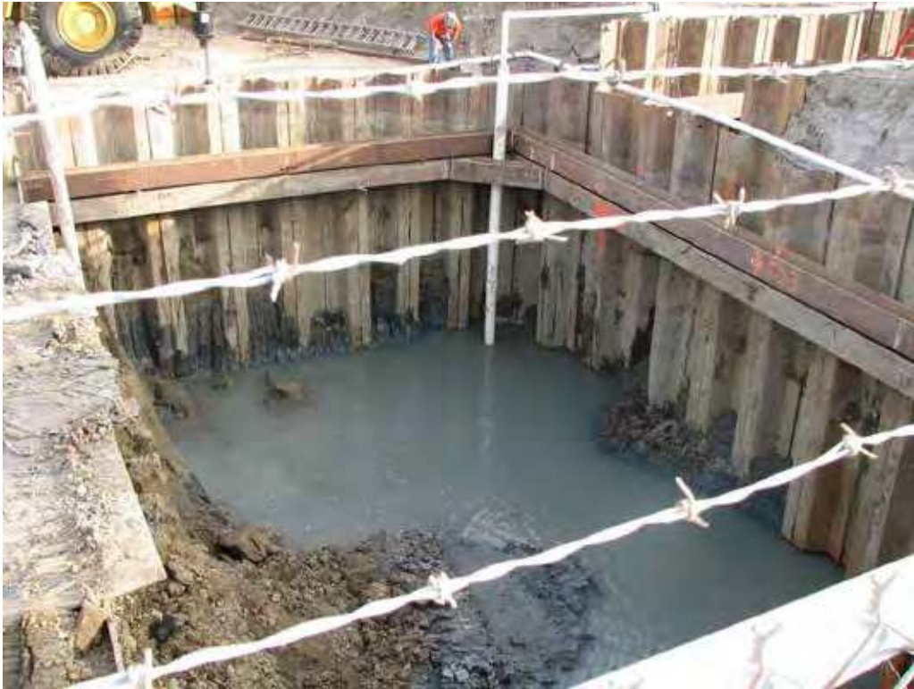
Photo 1 - Lift Station Excavation Flooded with Groundwater
