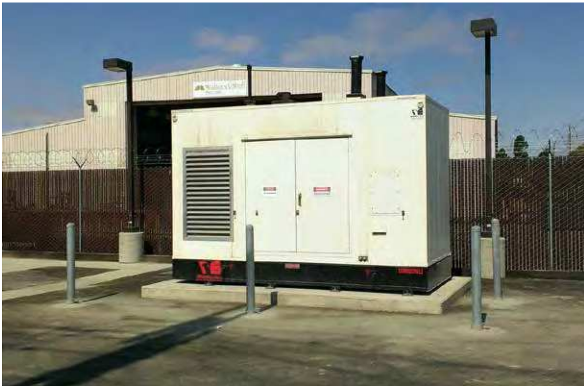
Photo 10 – Lift Station Standby Generator
