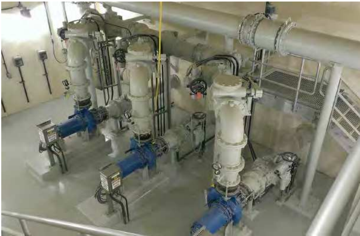
Photo 8 – Lift Station Drywell and Sewage Pumps
