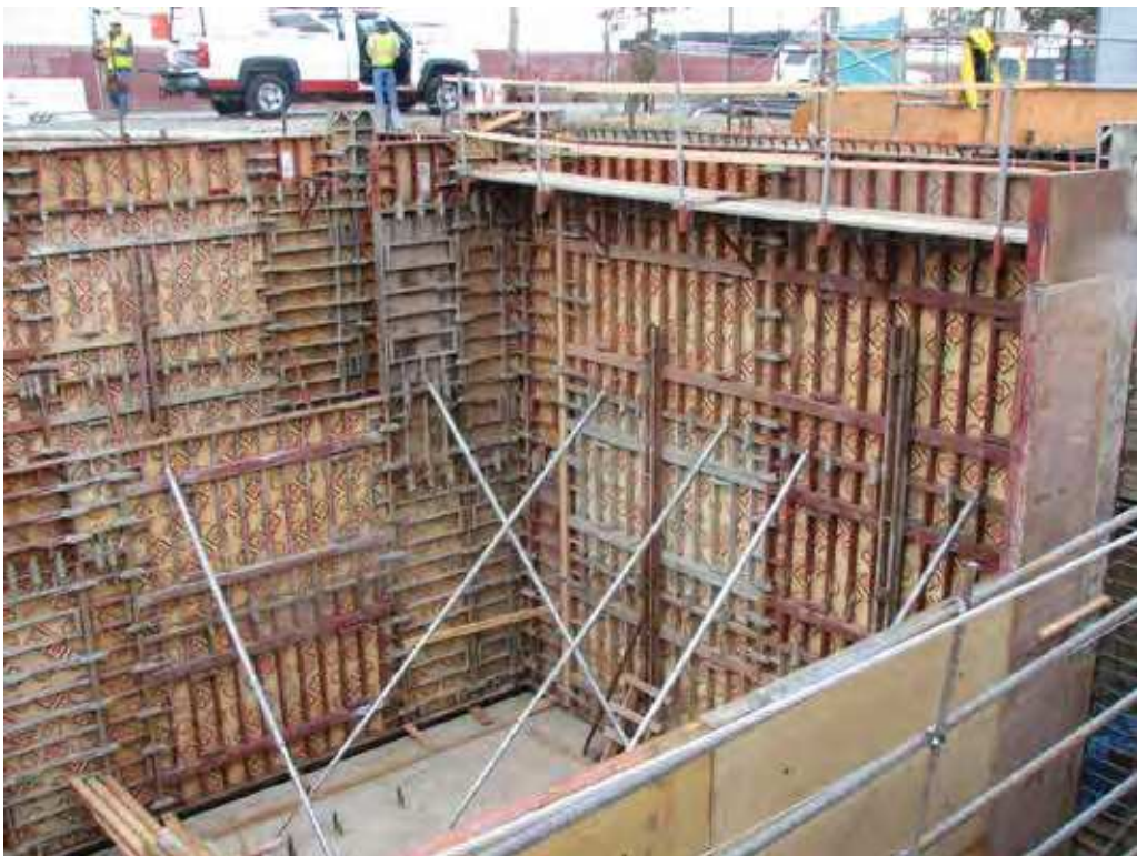
Photo 2 - Lift Station formwork and reinforcement placement.
