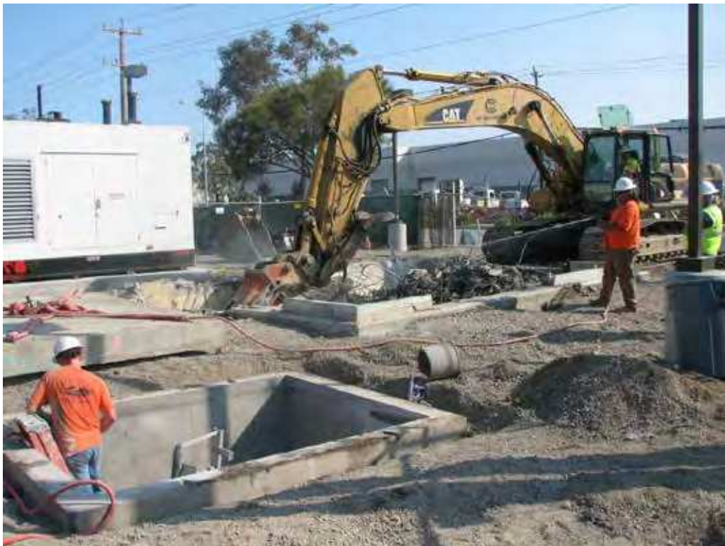
Photo 4 – Existing Lift Station Demolition
