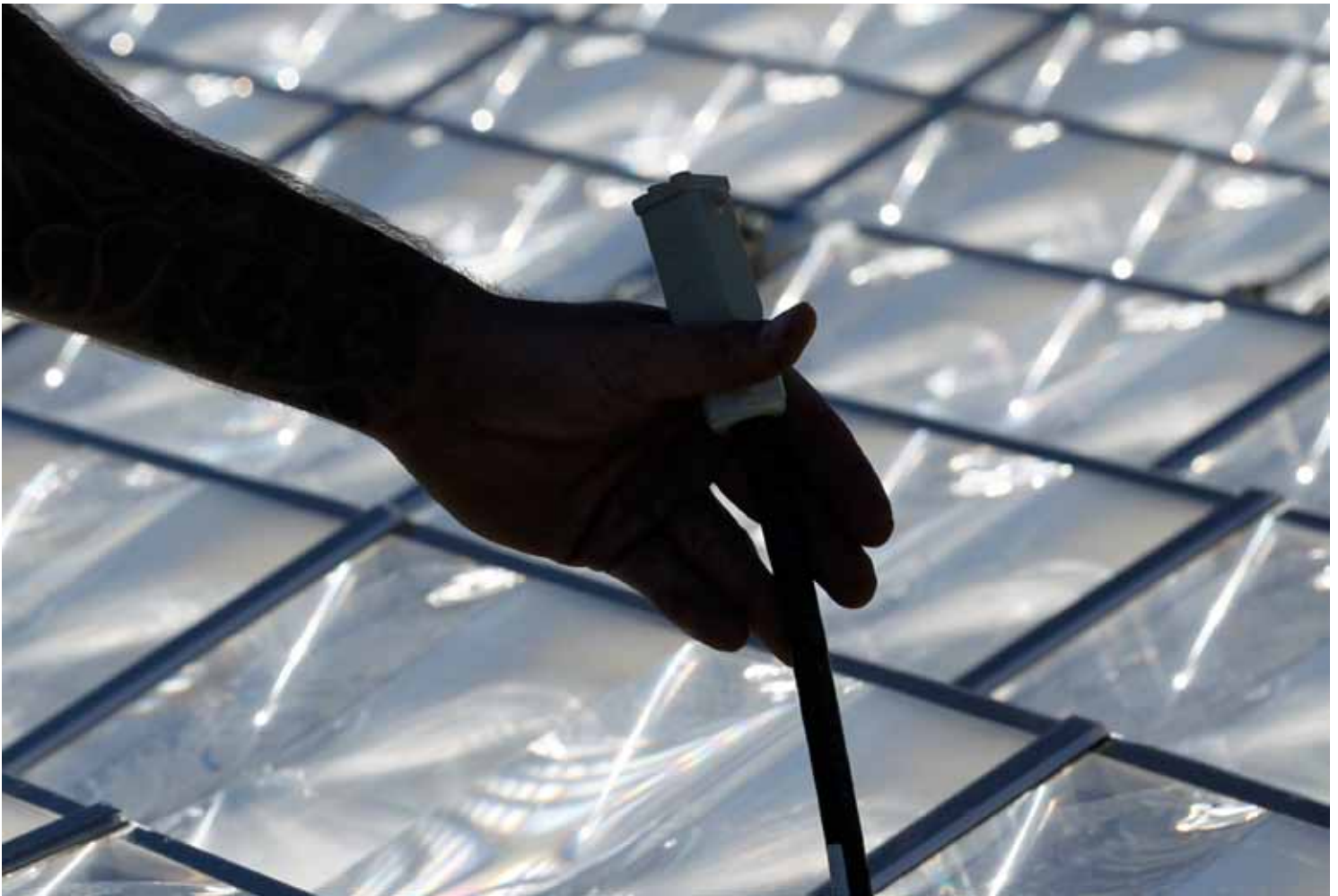
HIGH-TECH TOOLS: Workers assemble a Pyron Solar 90kWp DC CPV generating system that uses water to stay cool and track the sun in San Diego, California February 9, 2011. REUTERS/MIKE BLAKE
