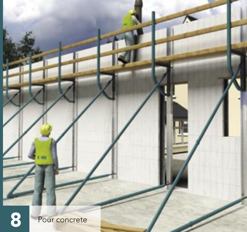
Adjust KORE Strut to ensure wall alignment
