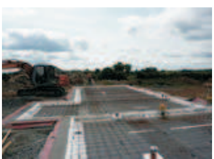
Install steel mesh & UF Heating Pipes
