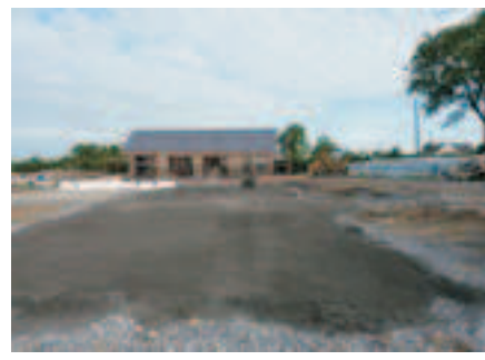
Limestone binding used to level off
