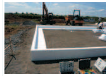
Install 1st layer of Ringbeam element
