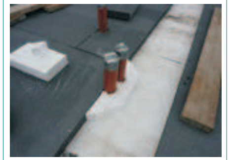
Insulate around pipes
