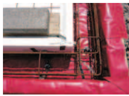
Install Steel in Ringbeam
