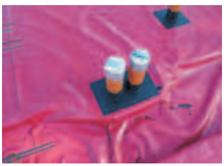
Install Radon Barrier
