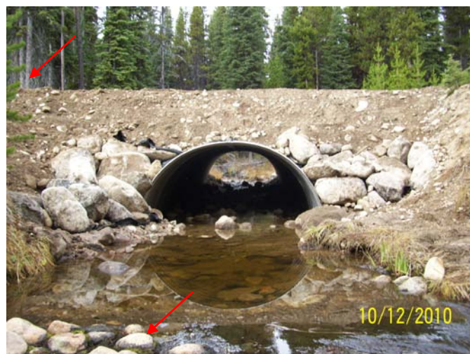
Photo 2: Completed new structure. Red arrows indicate same trees and same rock in photo 1 above.
