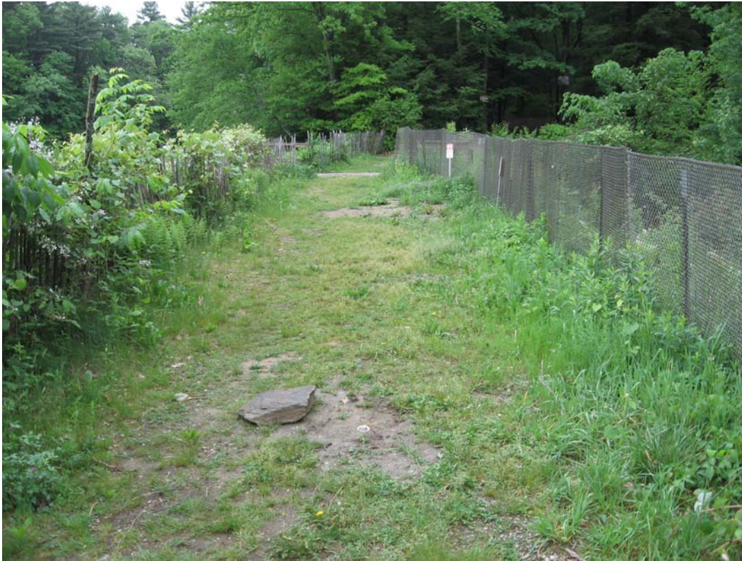
Photo 007. Crest looking right with piezometer location identified by stone
