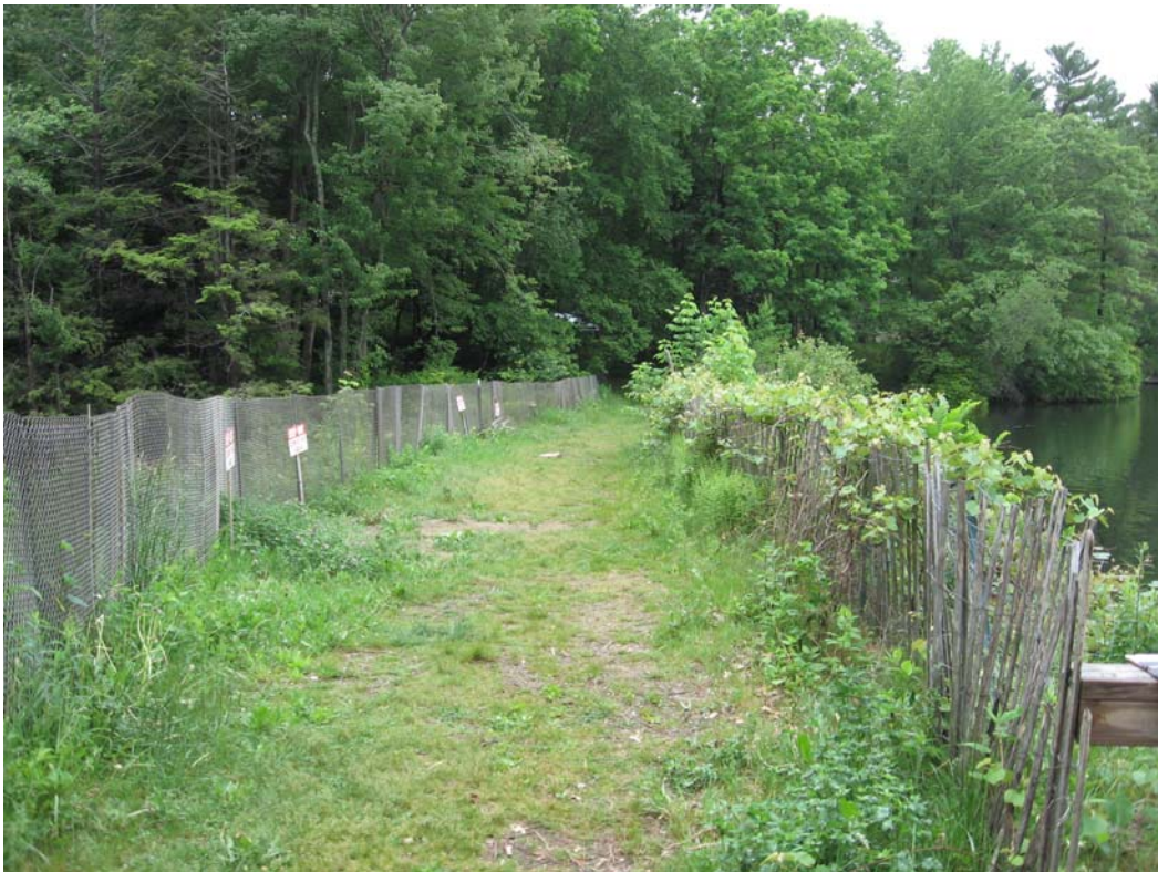
Photo 002. Standing on spillway looking right along crest
