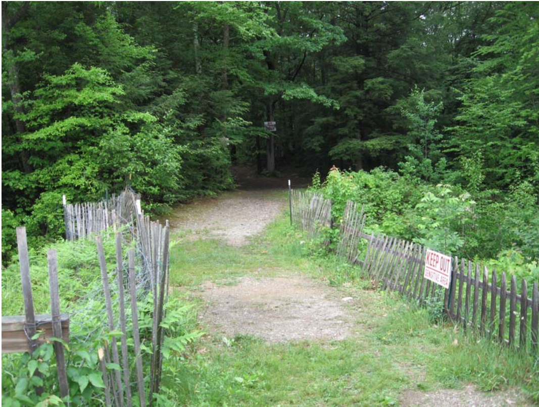
Photo 001. Standing on spillway looking at left abutment
