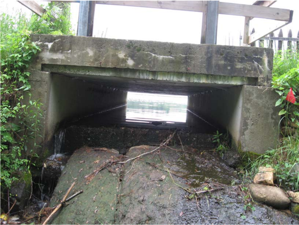
Photo 003. Spillway downstream opening
