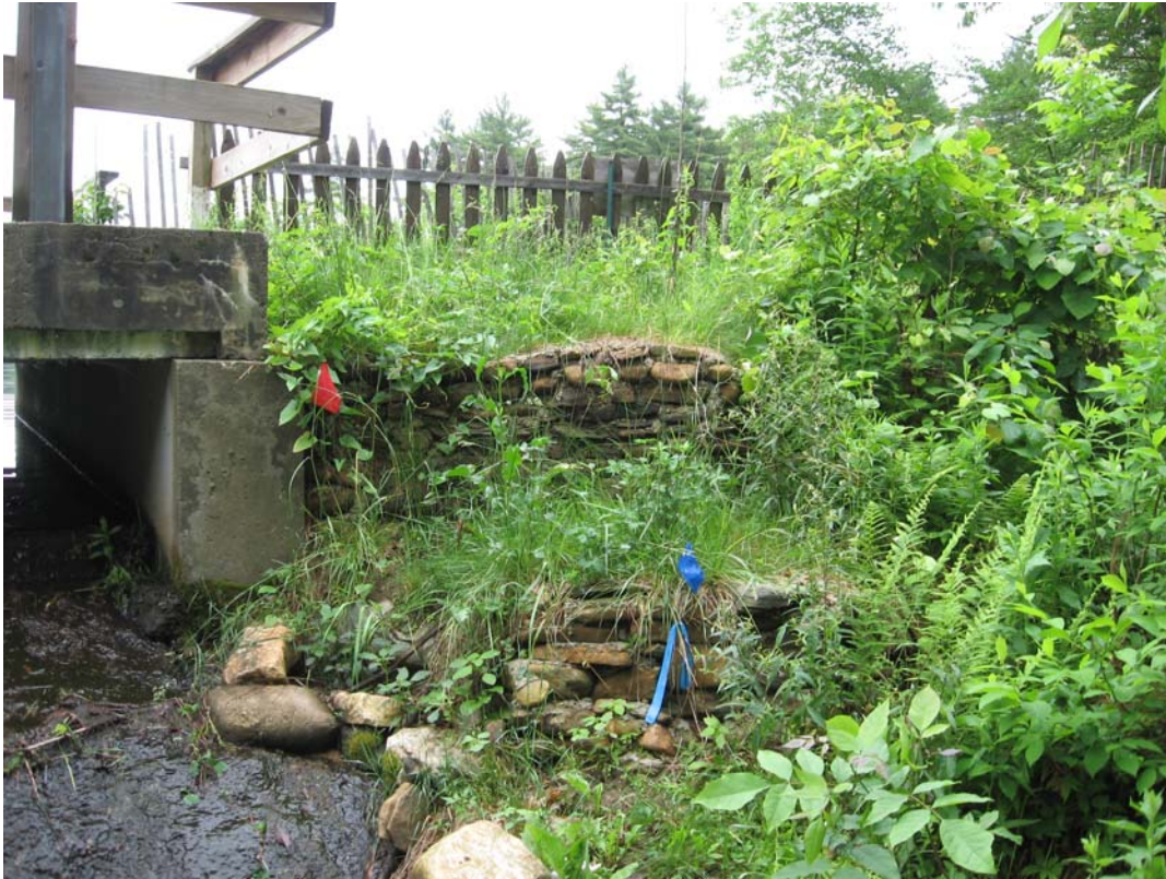
Photo 005. Right of spillway outlet
