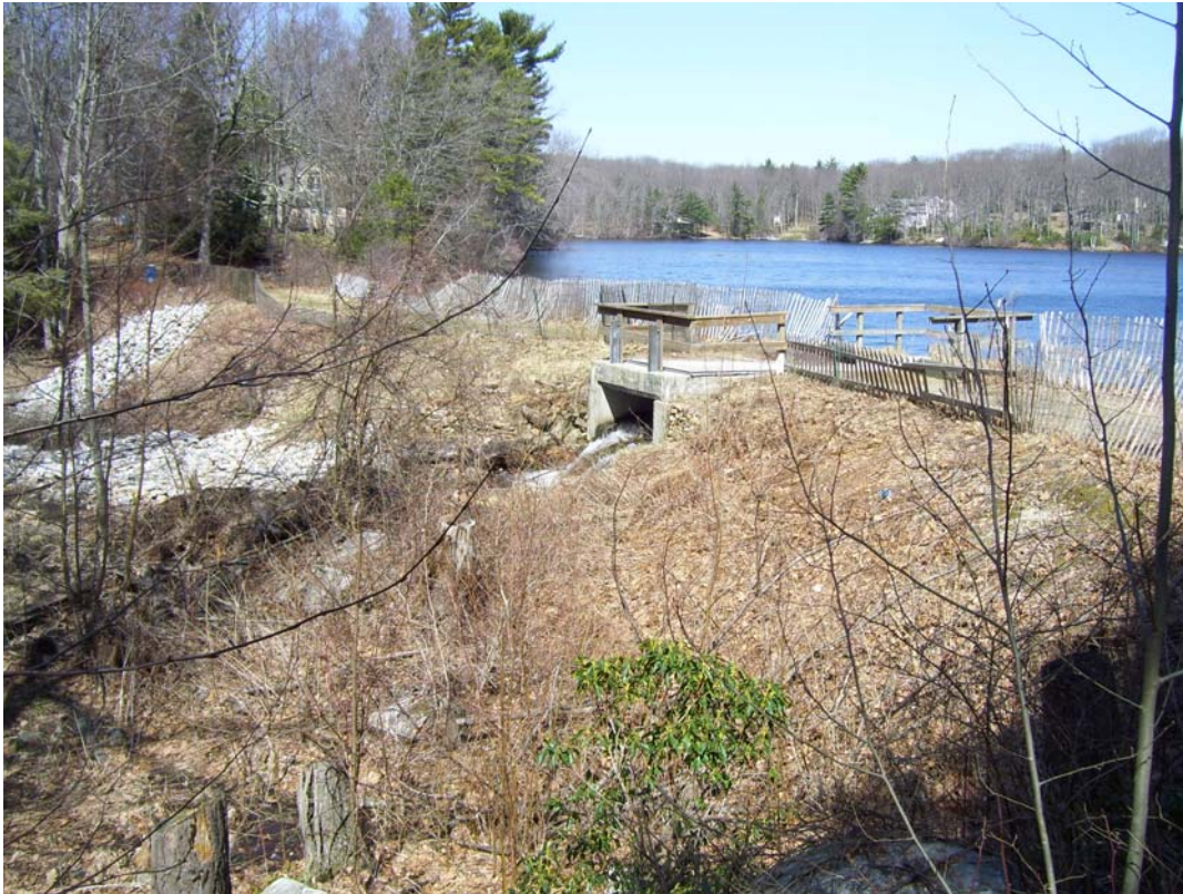
Photo 011-R. Downstream face from April 2008 Inspection
