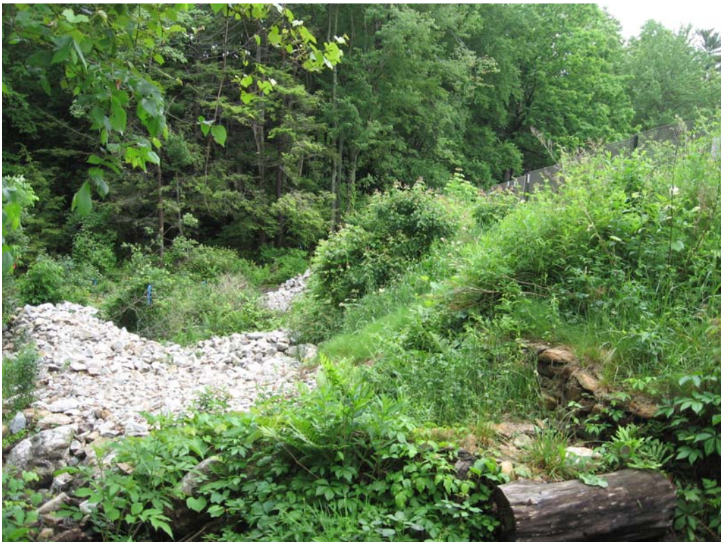
Photo 006. Downstream face looking right
