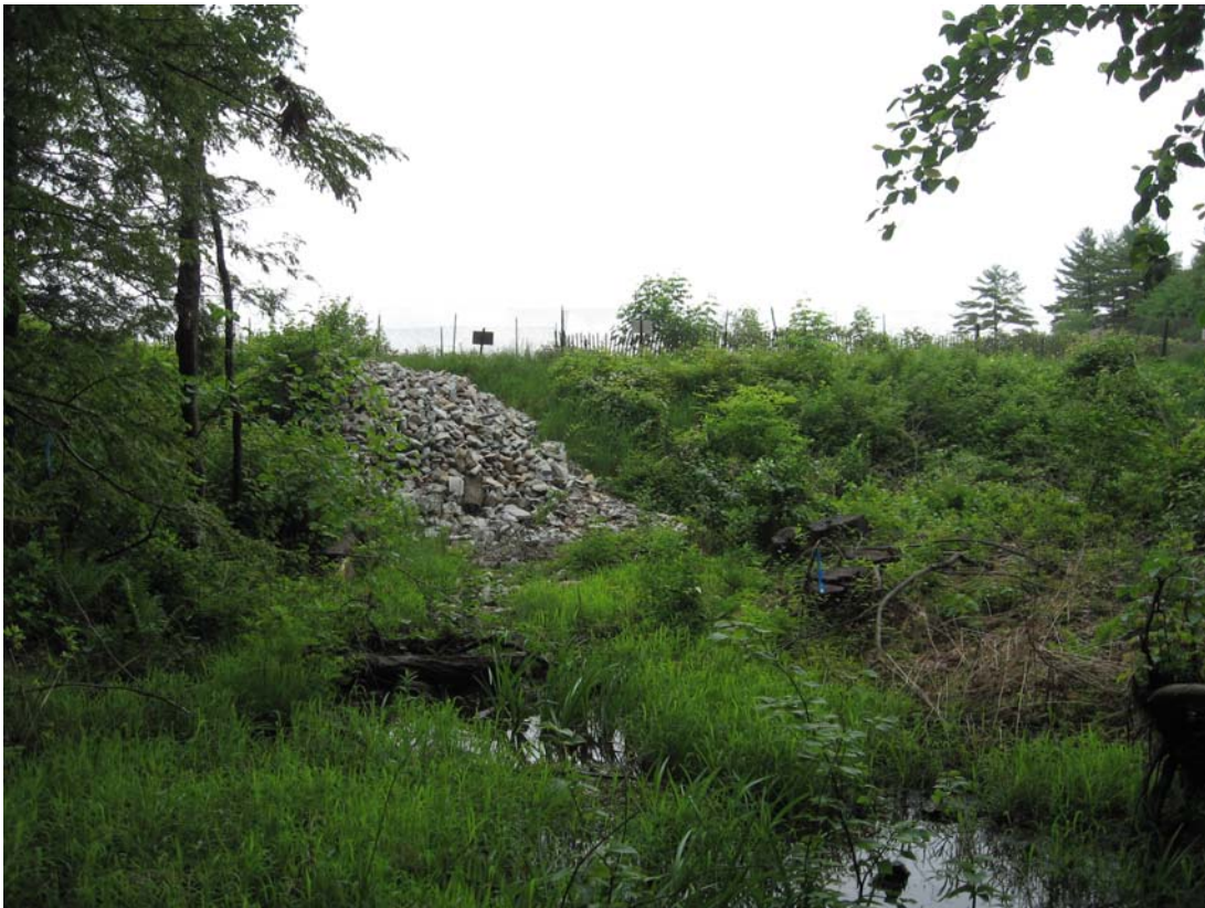
Photo 010. Downstream face with apparent out spillway outlet left of center
