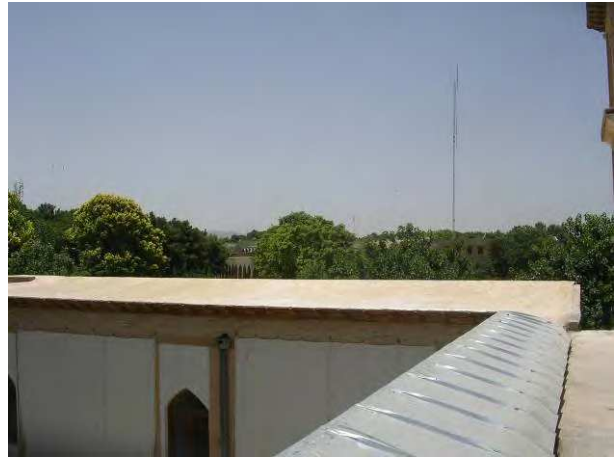
The roof is currently under repair, after it collapsed last May ('07)
