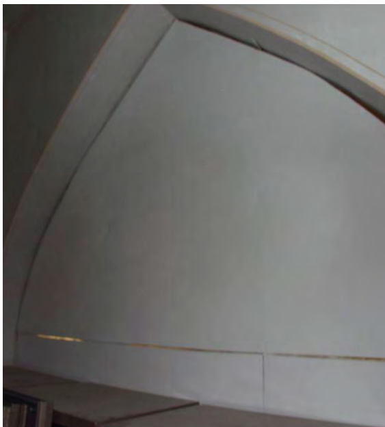
Arched windows fitted with a cut-out to shield sunlight
