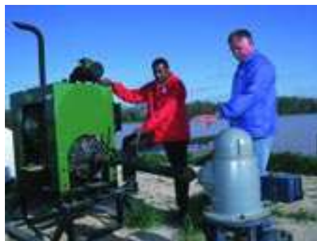
Tailwater recovery system
