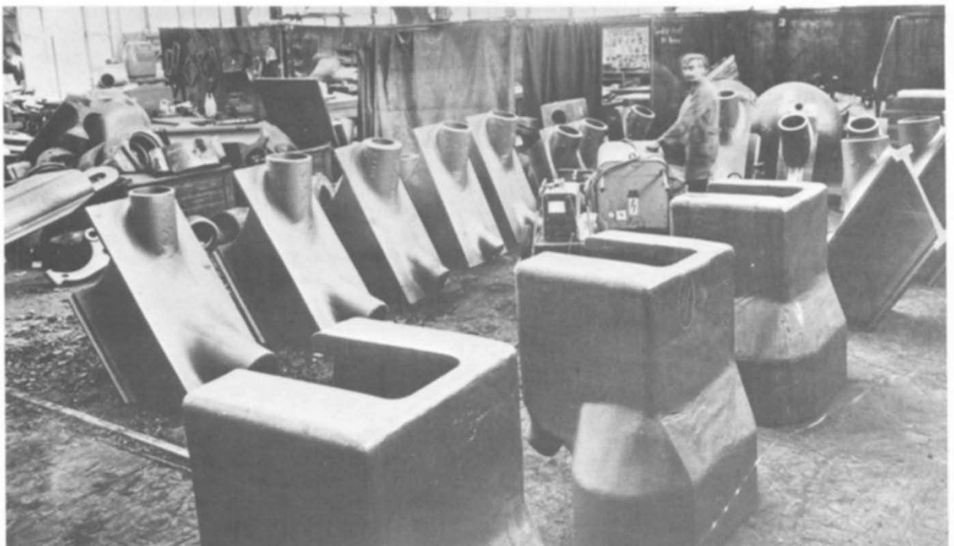
Figure 8—Ultrasonic testing of nodes of main girders in the Beaubourg Centre
