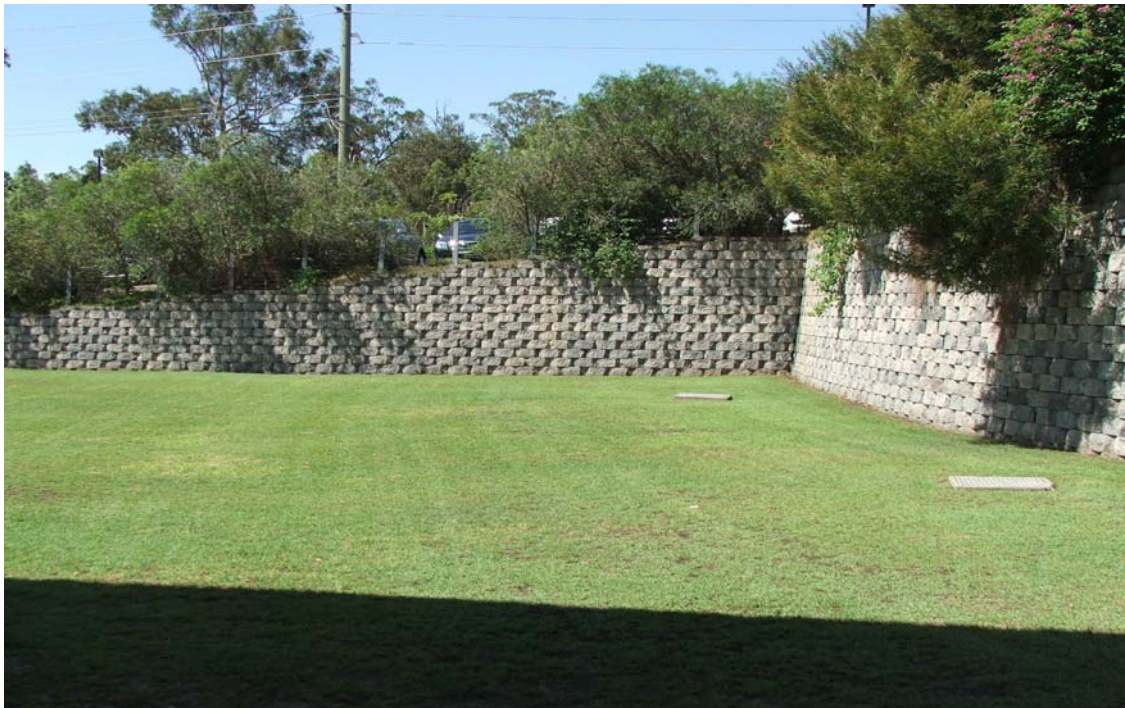
Figure 5: Location of hydrotherapy pool looking towards the New England Highway. Note the retaining wall. Source B Barrie 2010.
