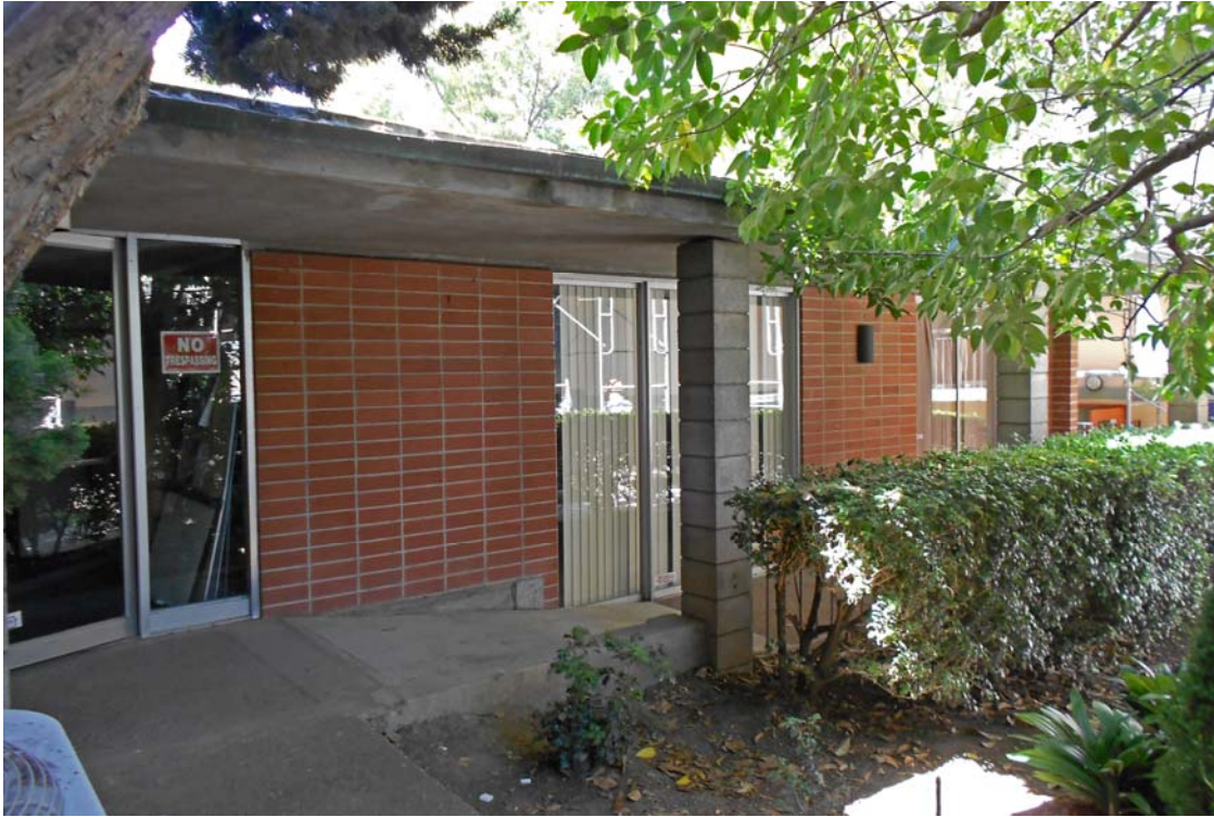
27) Educational wing north wall. View south.
