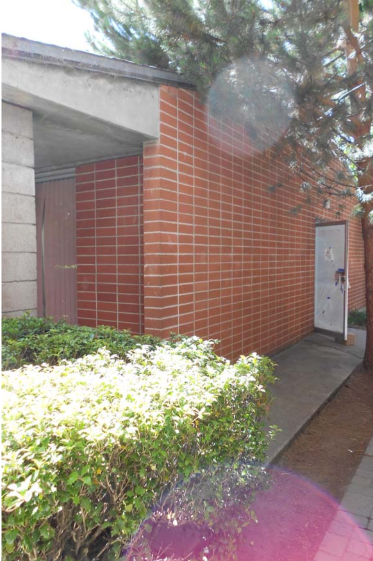
30) Educational wing west wall. View southeast.
