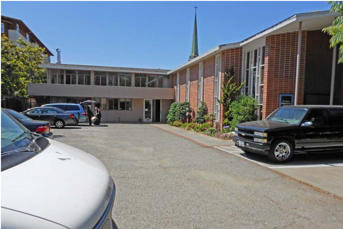
4) 1948 building: Administration wing (left); Sanctuary (right). View south.
