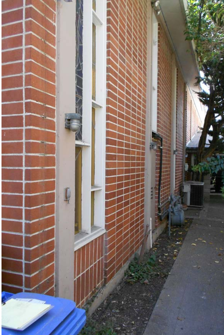
8) Sanctuary west side. View south.
