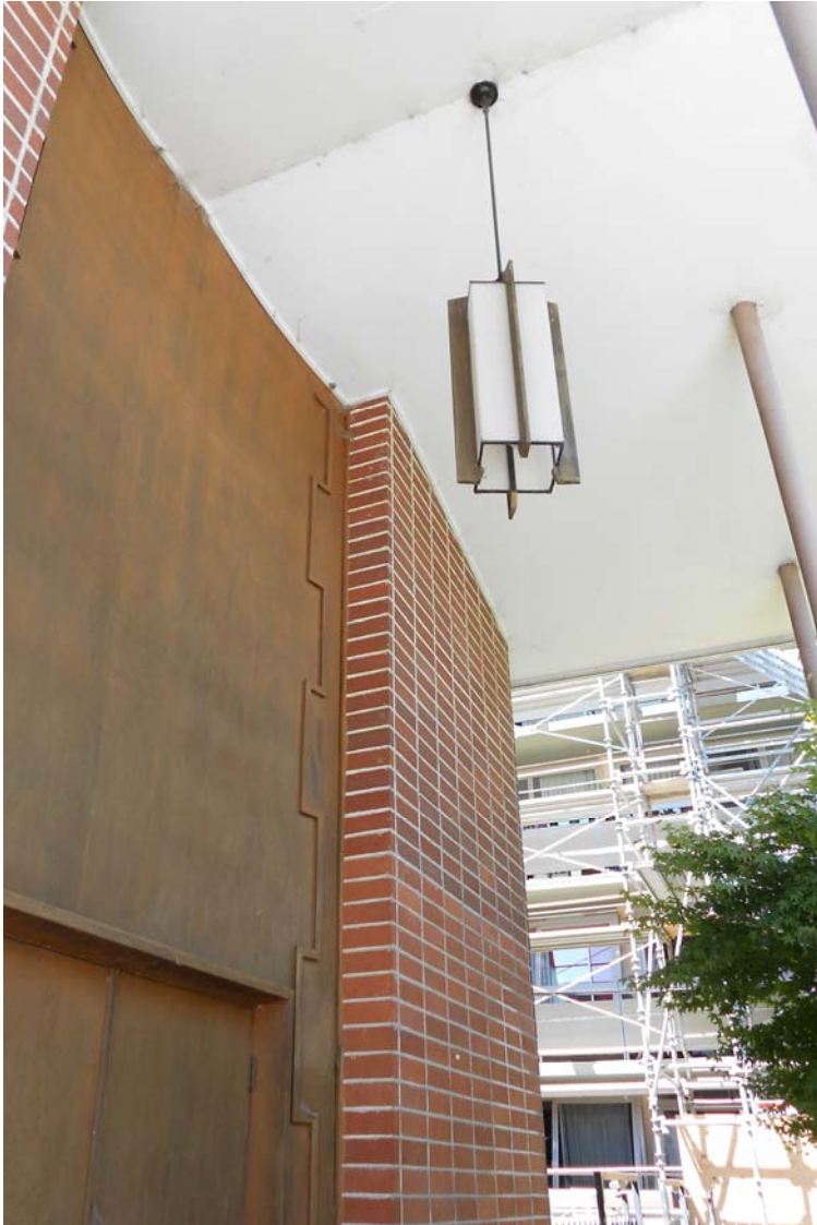
12) Sanctuary entry with wood door area and hanging lamp. View west.
