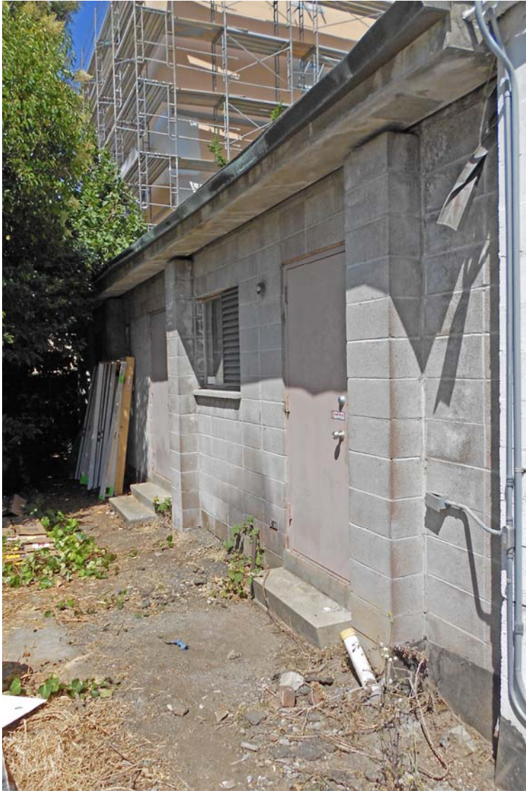
26) Educational wing rear wall. View west.
