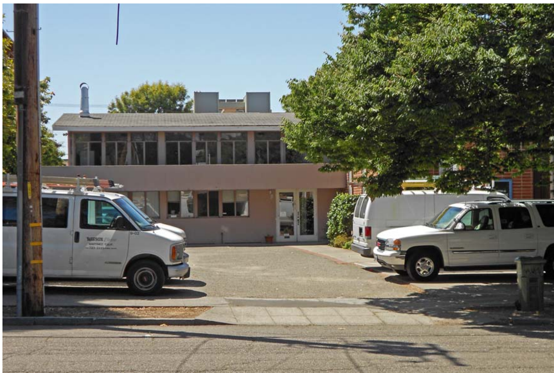
18) Administration wing. View south.
