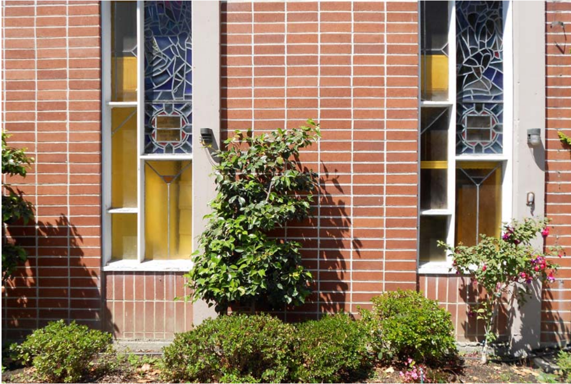
9) Sanctuary east wall detail. View west.
