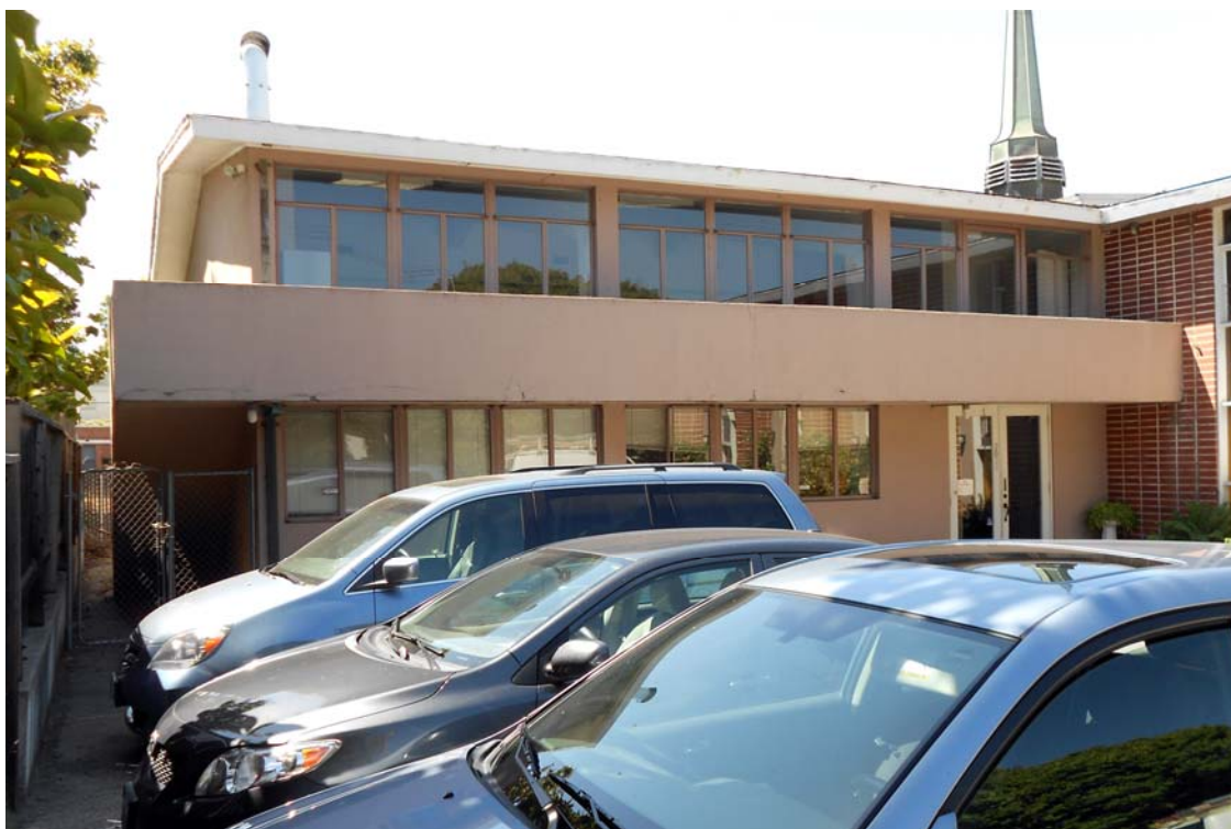
19) Administration wing. View south.
