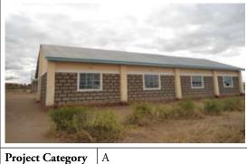
roject Status Complete and in use Comments: The materials used are of good quality and the workmanship is commendable. The foundation, walling, roofing and fixing of windows and doors are well done. The windows and doors are fitted with good coplars. The foundation is well set, walling well done with good quality stones and the roof is well set with facia board fitted. The overall project implementation is well done with
