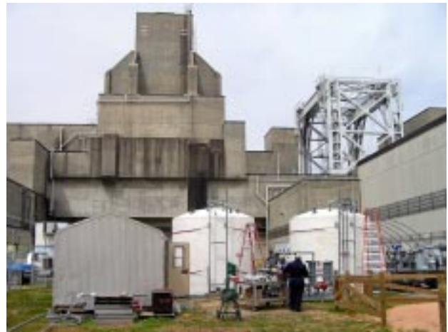
Electrical resistance heating project at C Reactor
