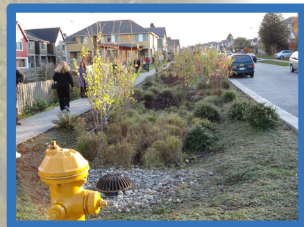
A photograph taken during the Seattle Field Trip to review the High Point Project's natural drainage systems.
