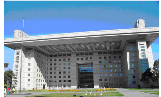
Administration Building at Beijing Normal University
