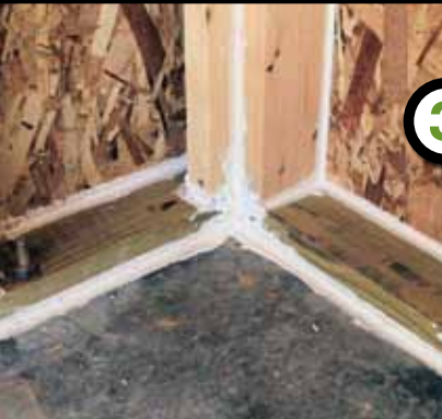
Caulk-sealed bottom plates
