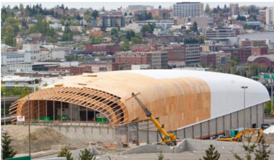
The curved roof, sheathed with fully sanded plywood, is streamlined like the aerodynamic surfaces of an automobile.
