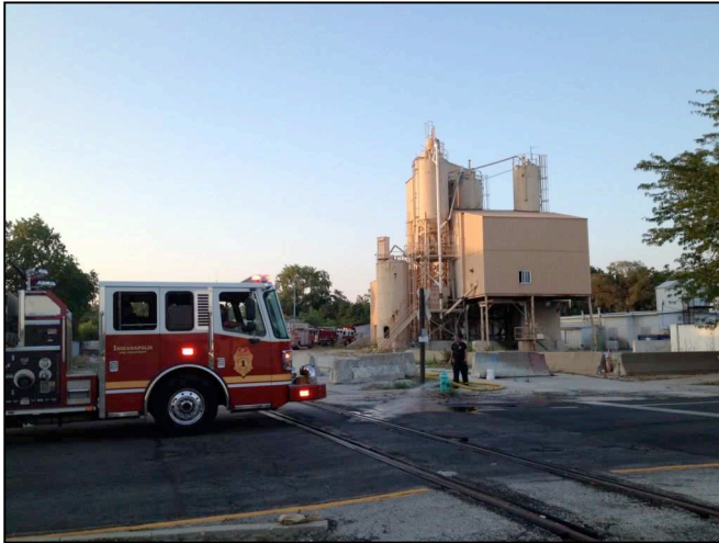
Hydrant pressure tested at working fire in RWELLS area
