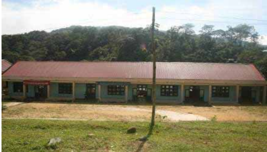
Photo: Primary school of Dak Man commune, repaired with financial support from DEC project
