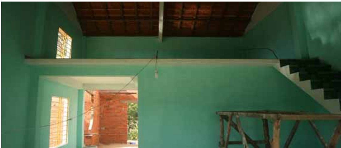
Photo: Model of flood and storm resistant house with reinforced tile roof, concrete room for storm and flood evacuation. (House of Mr. Bong, Tam Hai commune, Nui Thanh district)
