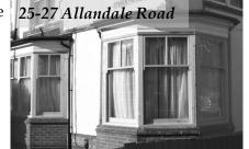
the original design and would be better still. Ground-floor timber windows recently installed to replace obsolete metal units at 25-27 Allandale Road show how well this can be done.
