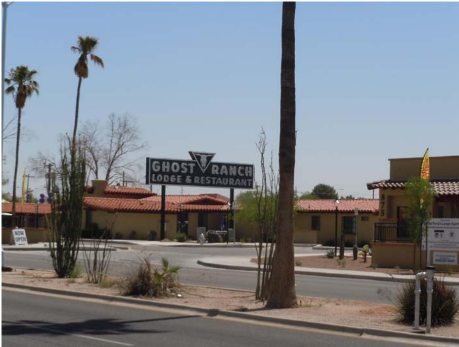
1. Original Building Group Approach to Ghost Ranch Lodge at Building Q and Sign X. View to Southeast. (Photo by Don W. Ryden of Ryden Architects, Inc., 2011)
