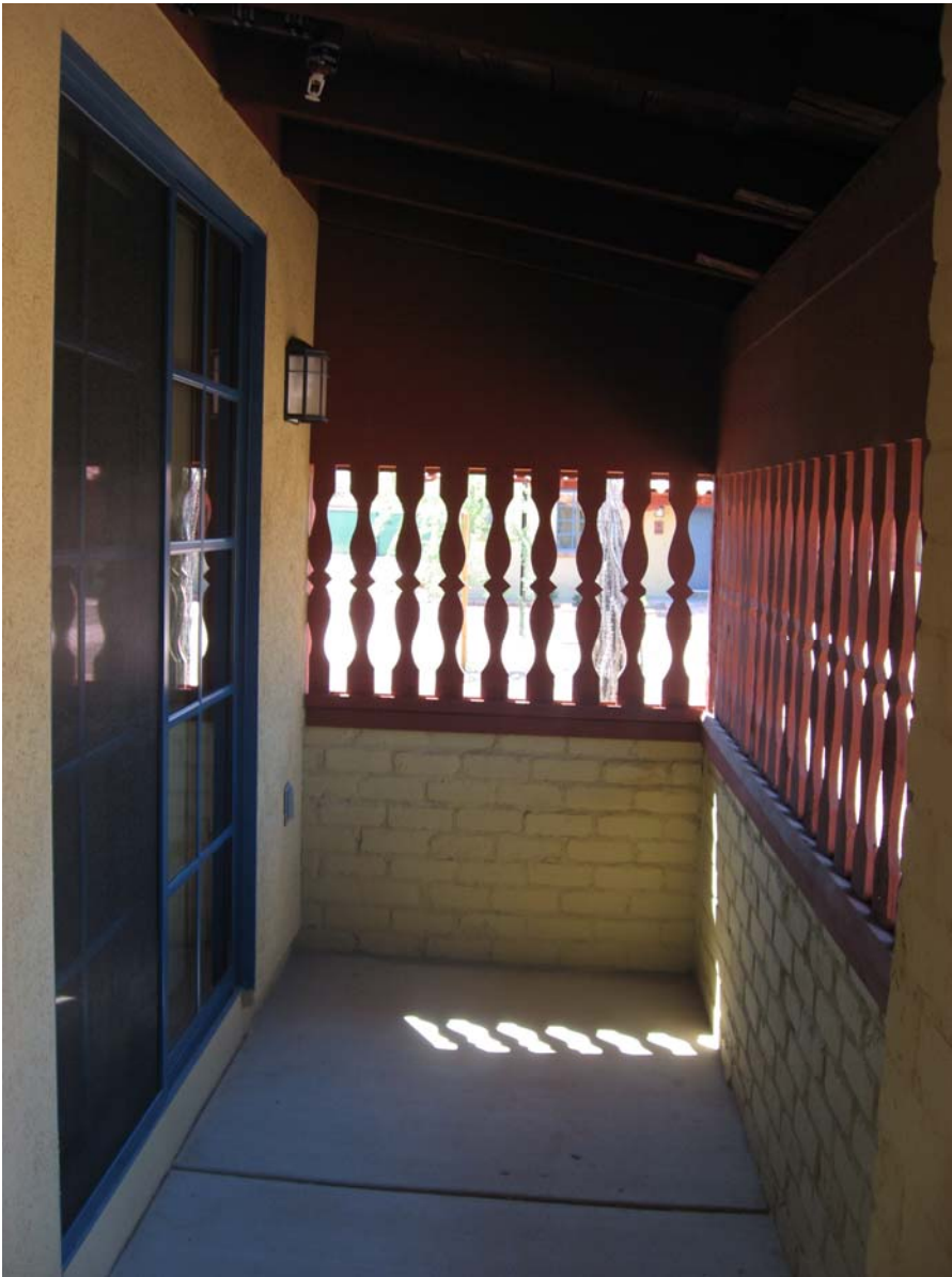
40. Original Building Group Recessed placement of the bedroom infill retains character of open carport in the form of a patio. (Photo by Don W. Ryden of Ryden Architects, Inc., 2010)
