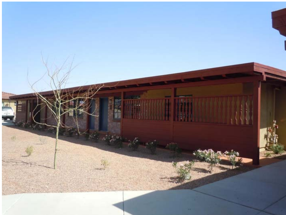
18. First Building Group Addition Spanish Colonial Ranch Style linear units (Building I) with covered walkway and end carports. View to southeast. (Photo by Don W. Ryden of Ryden Architects, Inc., 2011)
