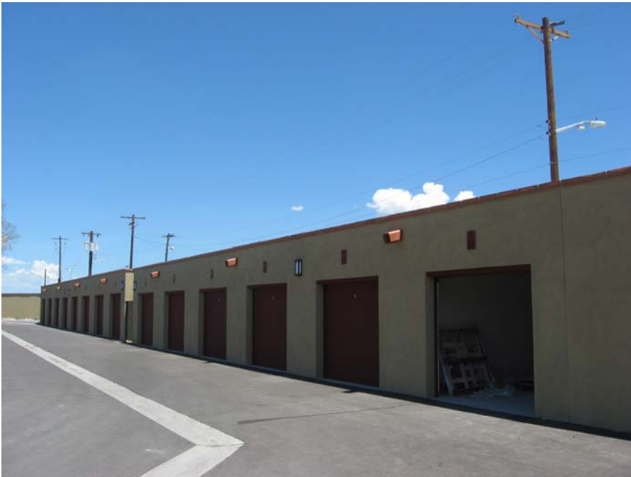
35. Fourth Building Group Addition New garages (Buildings 7 and 8) line the east edge of the property. They are unseen from the historic Courtyard AA. View to north. (Photo by Don W. Ryden of Ryden Architects, Inc., 2011)
