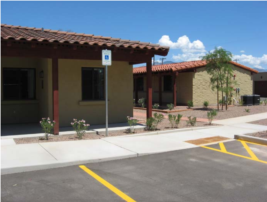
32. Fourth Building Group Addition The simple details and finishes of the new Apartment (Building 4) (foreground) defer to and complement the historic character of the Joesler-designed Building D (background). View to northeast. (Photog by Don W. Ryden of Ryden Architects, Inc., 2011)
