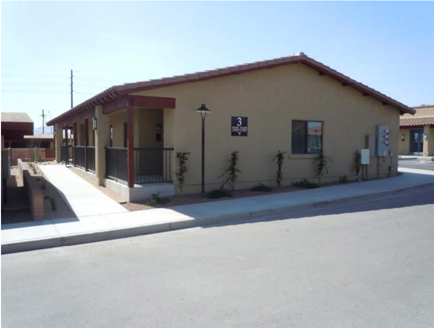
30. Fourth Building Group Addition The new, one-story Apartment (Building 3) is a simplified interpretation of the Joesler-designed duplexes. View to northwest. (Photo by Don W. Ryden of Ryden Architects, Inc., 2011)
