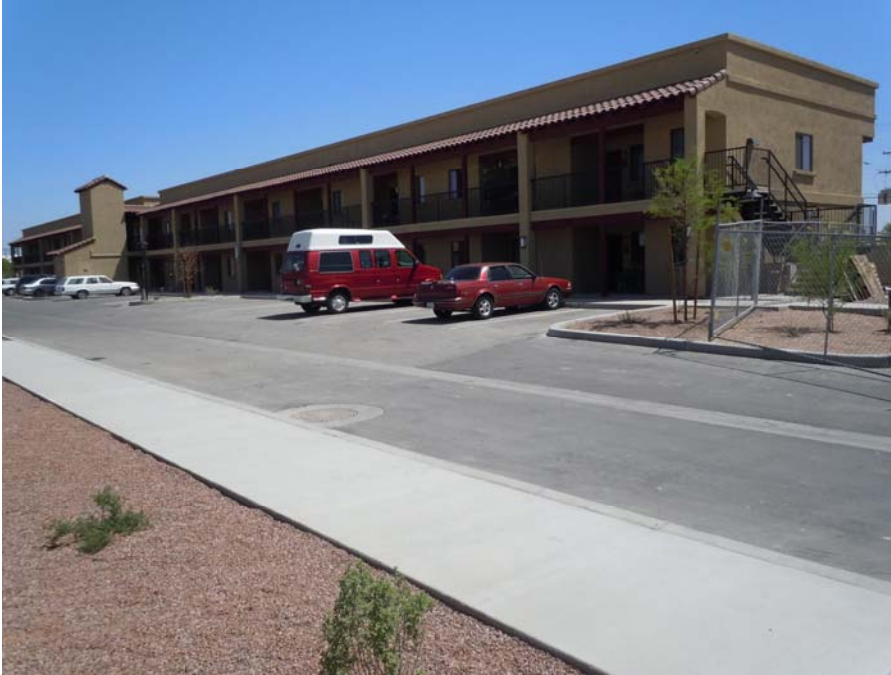
34 Fourth Building Group Addition The new, two-story Apartment (Building 6) stands at the rear of the property where its height has no adverse effect on the one-story historic buildings. View to southeast. (Photo by Paul C. Sikorski of Ryden Architects, Inc., 2010)
