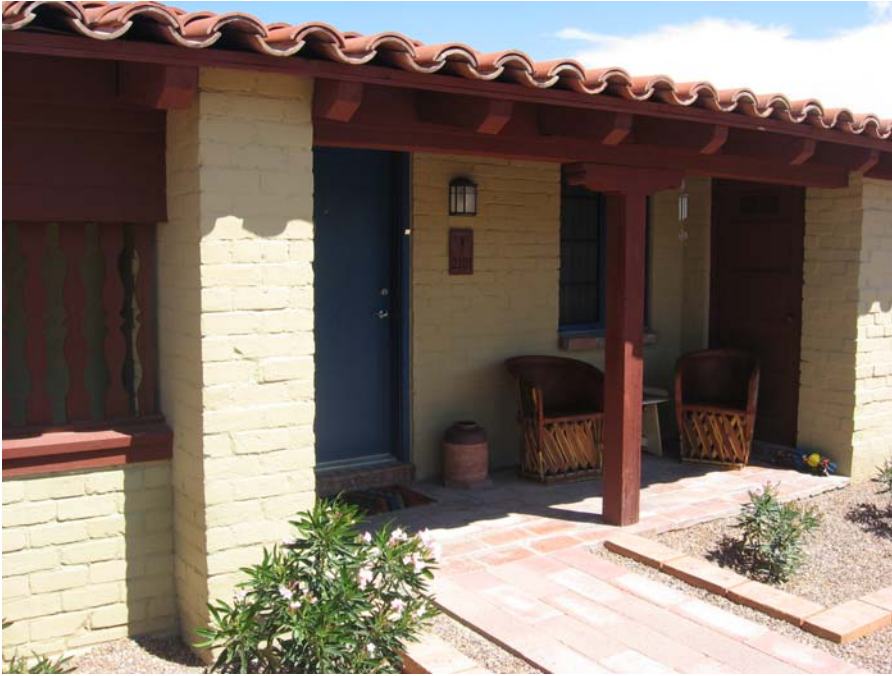
11. Original Building Group Rehabilitated entry porch at Building C. View to northeast. (Photo by Don W. Ryden of Ryden Architects, Inc., 2011)
