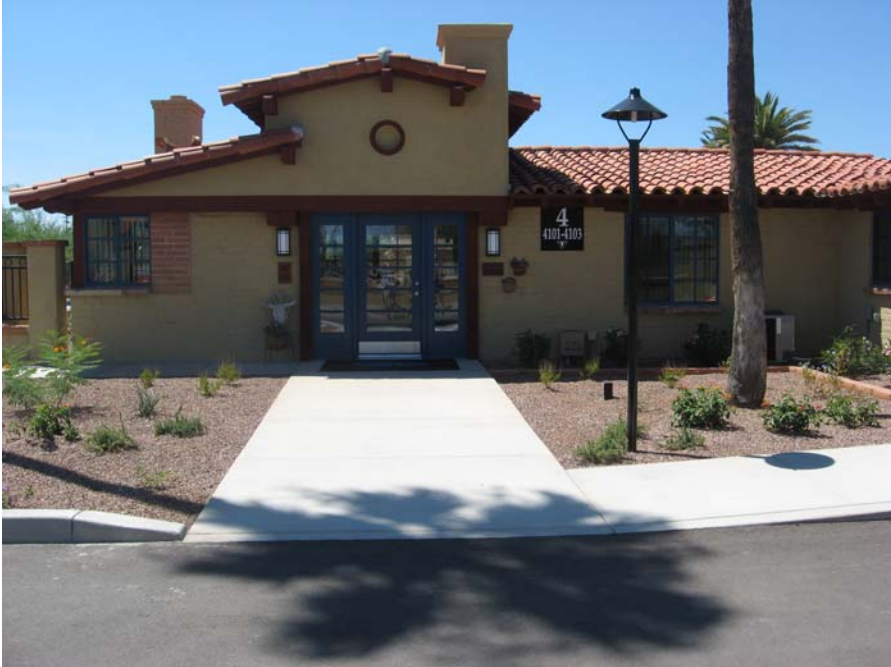
6. Original Building Group Entrance to rehabilitated Office Q. View to south. (Photo by Paul C. Sikorski of Ryden Architects, Inc., 2010)
