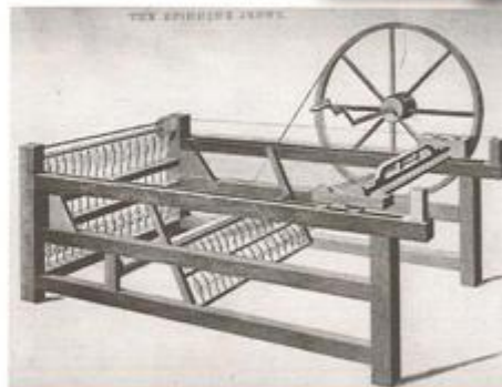
A diagram of c. 1750 showing the Spinning Jenny.
