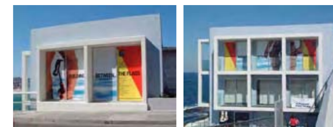
Building signage with complete installation (Client – Easton Builders for Bondi Icebergs Club, Bondi Beach, Sydney)
