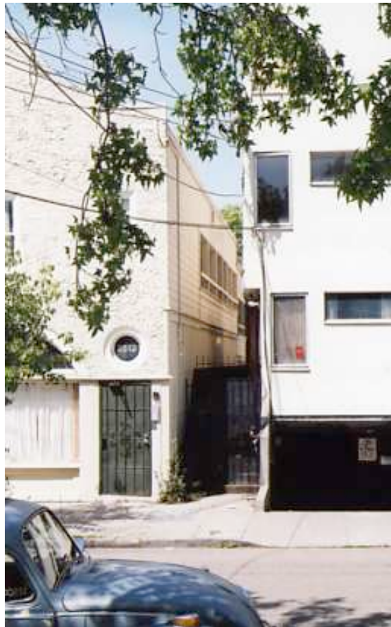
Fig. 12 Oblique view of north wall, May 2009
