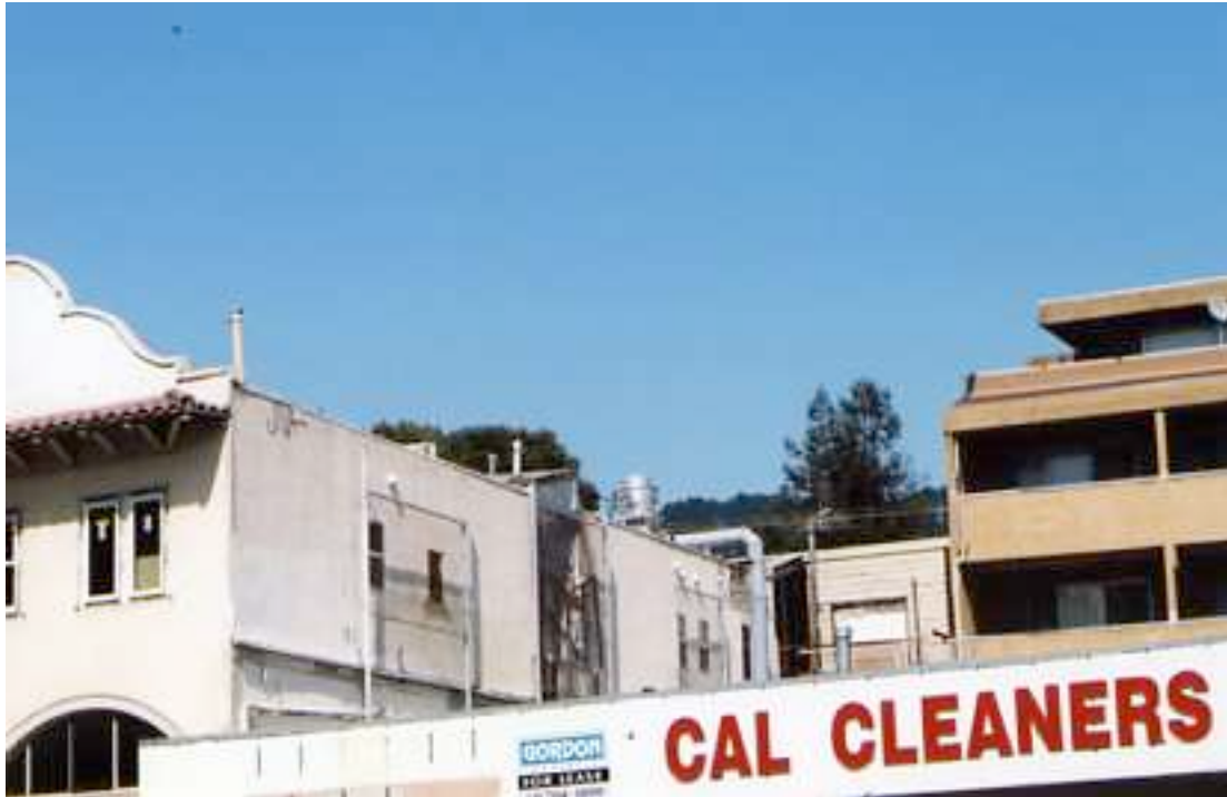
Fig. 5 Oblique view of one of the south walls, May 2009
