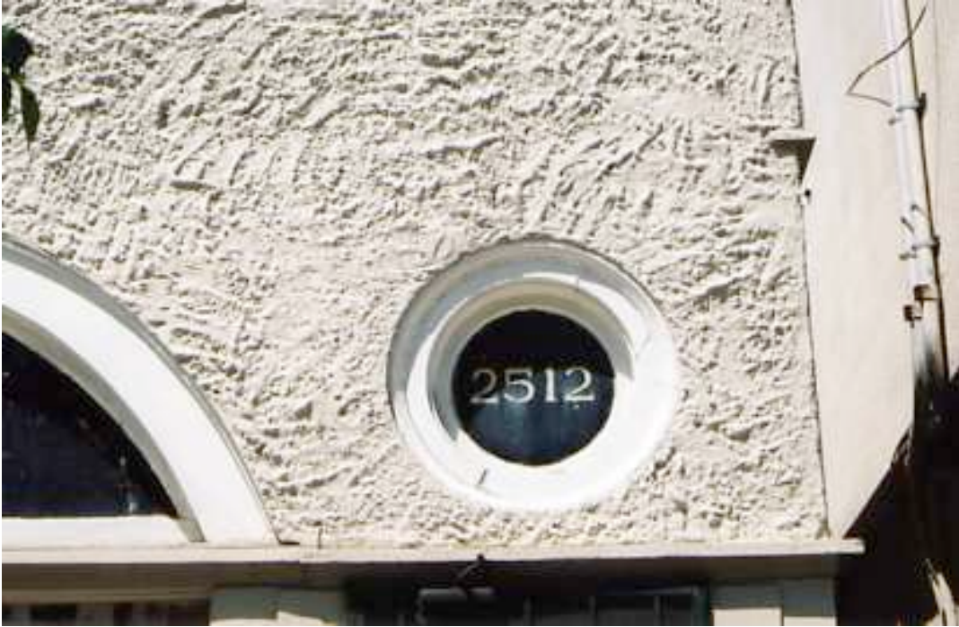
Fig. 11 Porthole window on regent Street façade, May 2009
