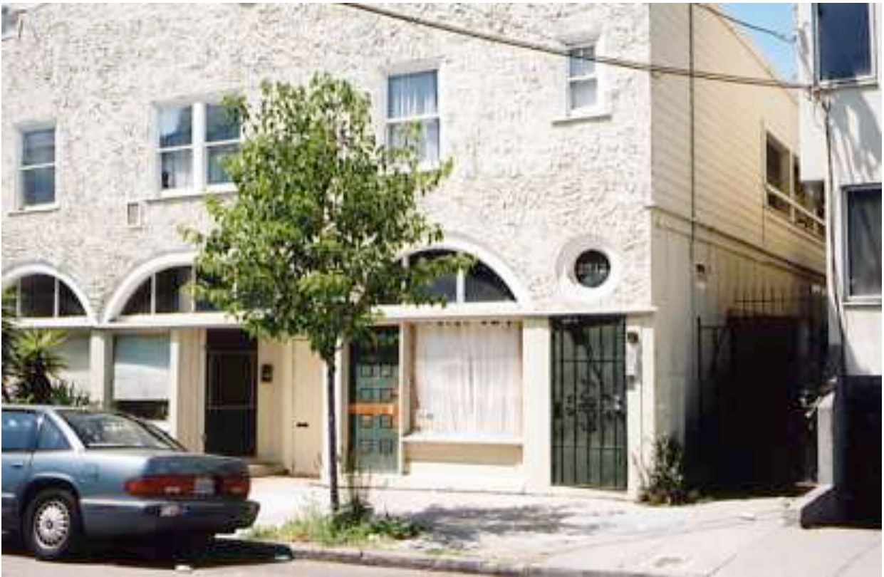
Fig. 10 Windows and doors on Regent Street façade, May 2009
