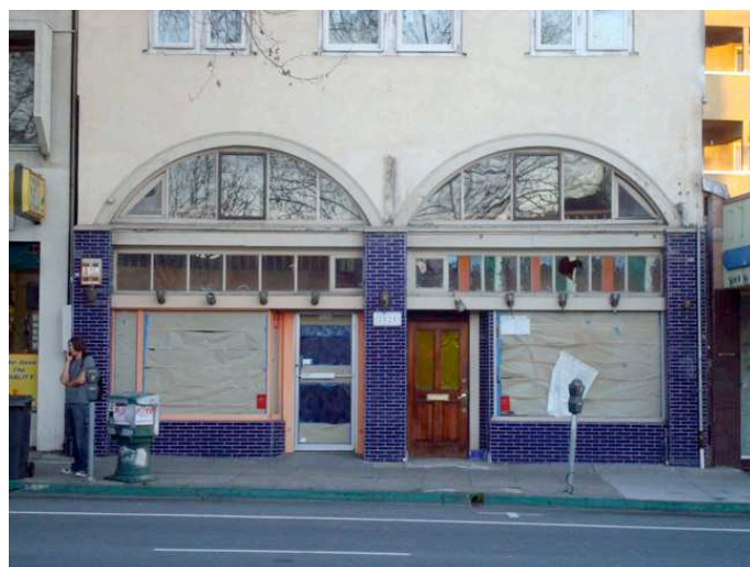
Fig. 2 Lower portion of Telegraph Avenue façade, March 2009
