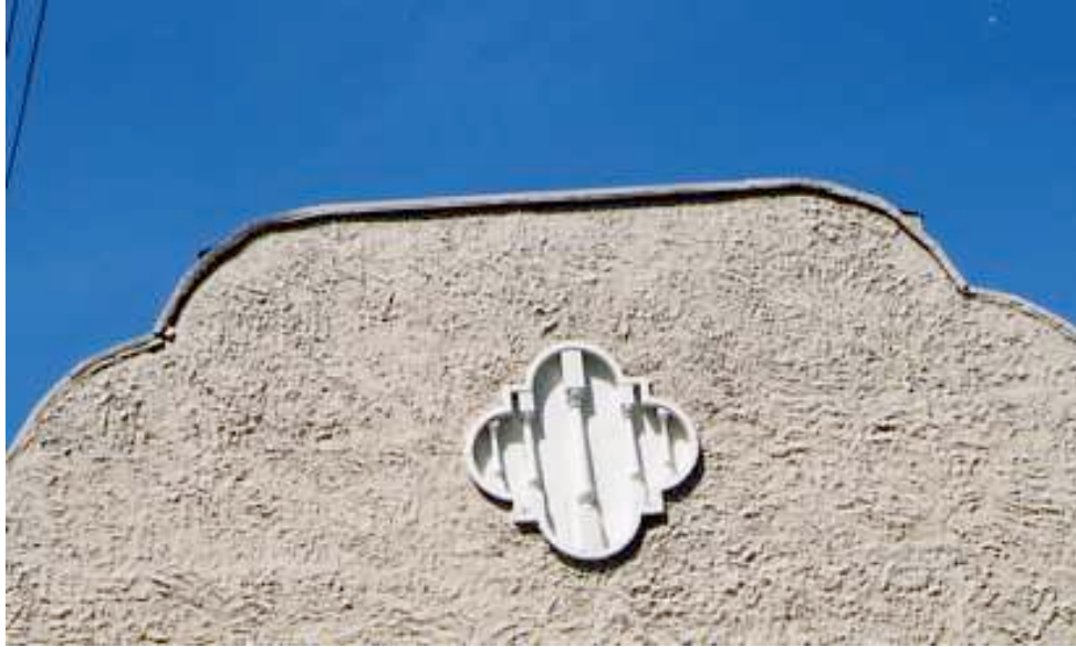
Fig. 13 Quatrefoil detail on regent Street façade, May 2009
