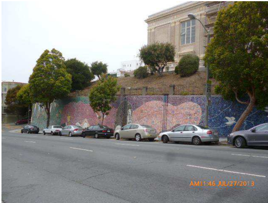
Figure 10 – North side of Fell Street east of Pierce Street
