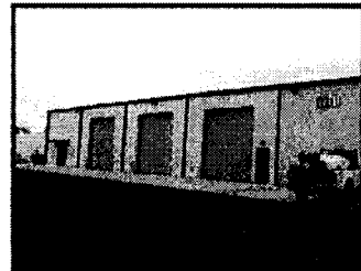
Brazoria County Pct. 4 Shop Building
