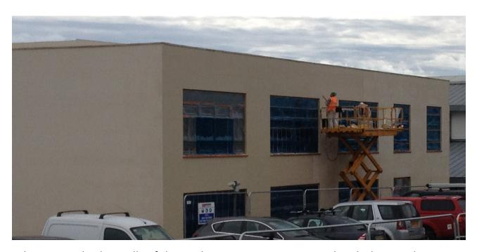
The rear and sides walls of the Sixth Form Centre are coated with the weatherproof render and are now close to completion. Plans for the internal furnishings and fittings are now been finalised. Examples above are representative of styles chosen rather than the colours selected.
