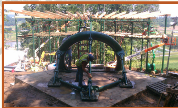
Finishing touches are made attaching this thing to the collaborative dead man and micropile anchors below...
