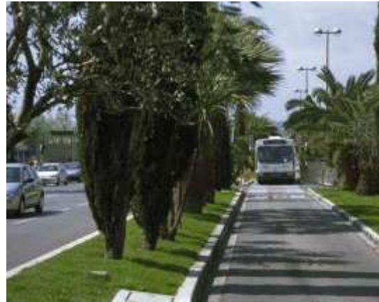
Figure 4: dedicated bus lane
