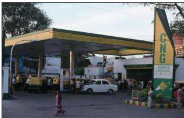
Figure 28: CNG fuel station, Delhi, India
