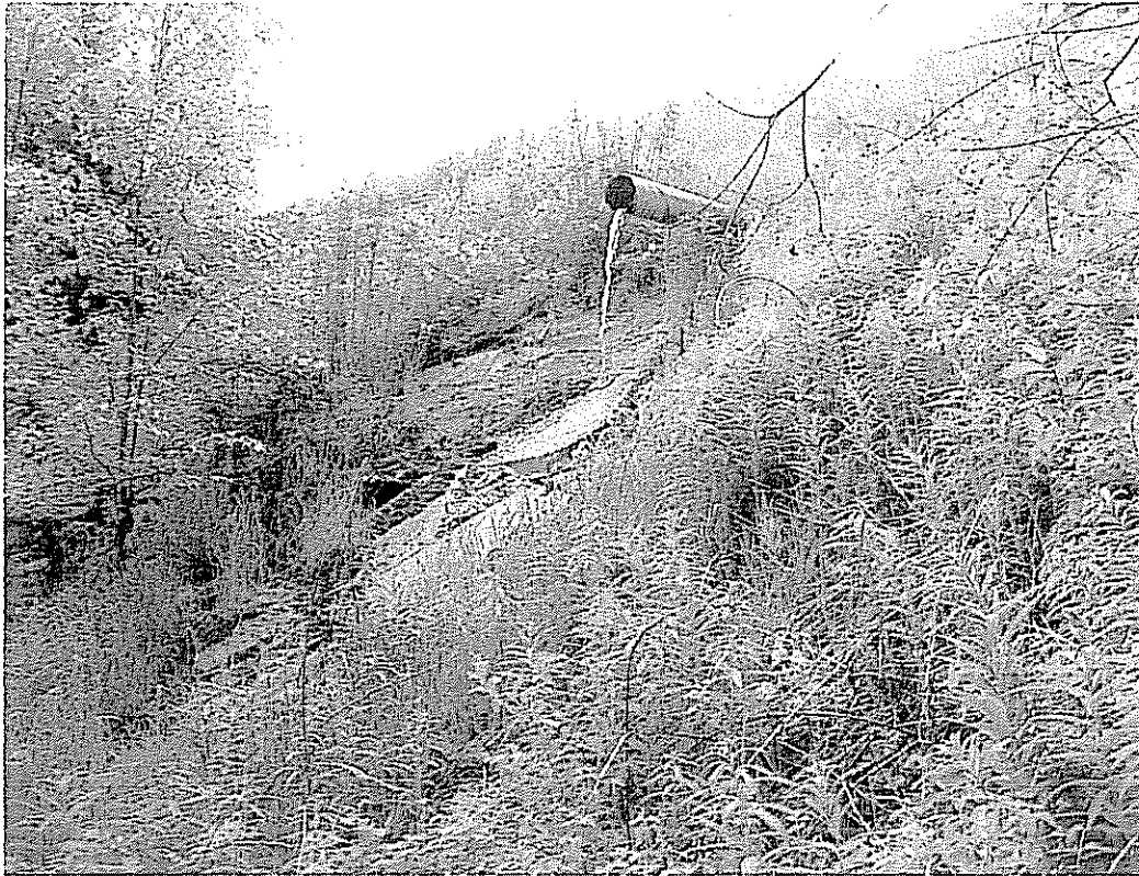
Stream section begins from culvert outfall in fill at top of gully below Hillside Park.
