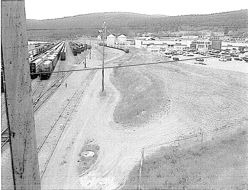
Stream flows into ditches that are culverted under Canadian Tire and then enter storm sewer at the railway tracks.
