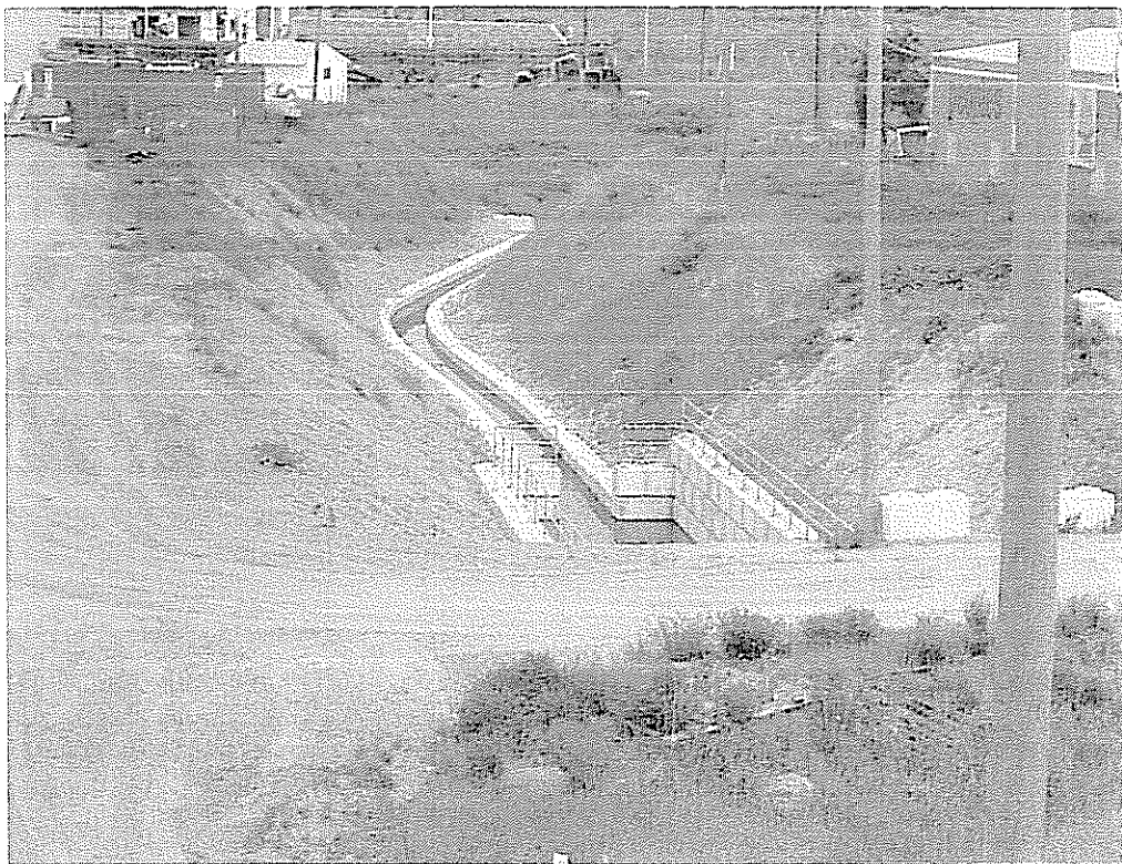
Storm sewer ends at San Jose River
