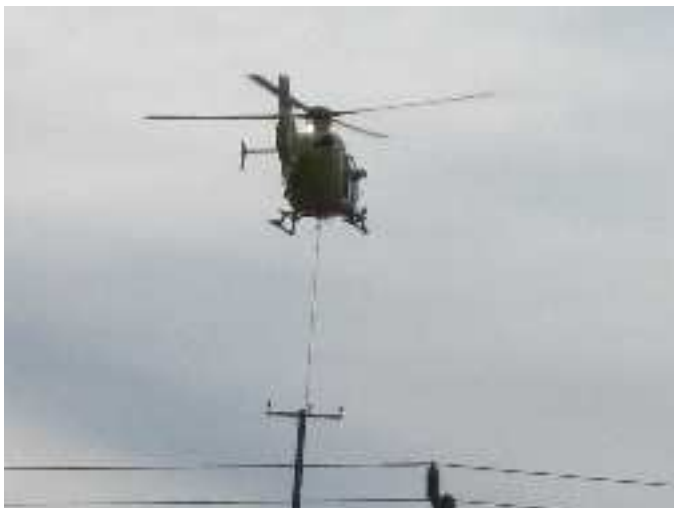
Helicopter used to install new poles
