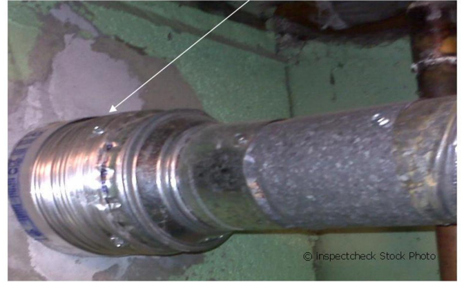
Flue / Vent Pipe - INSTALL FLUE LINER
