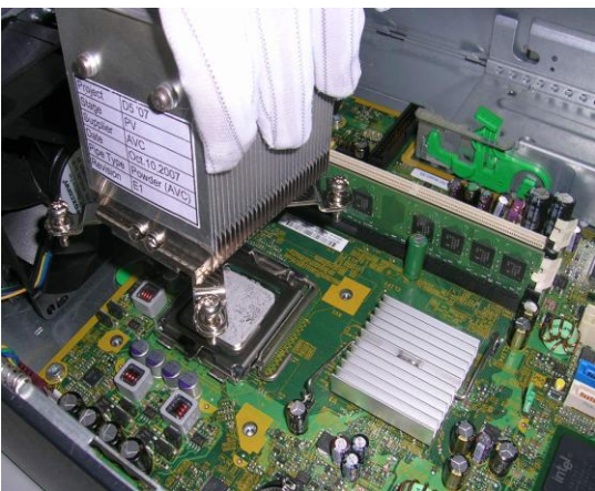
Figure 11: Remove Heat sink from PCA
