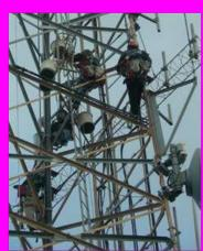
ITA tower standards. We also tidled up the tower and improved its loading by removing unused cable cords and antennas, ensuring that the tower can support its tenants, two FM broadcast antennas, three Cricket cellular phone antennas, two high performance wireless research and educational network microwave anten-
